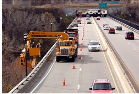
Figure 3: A bridge inspection using truck & boom.
