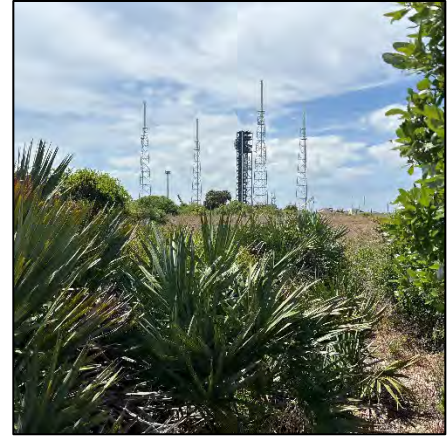
Figure 7-18. Overview of 8BR04011, facing west from ST N700E725.
