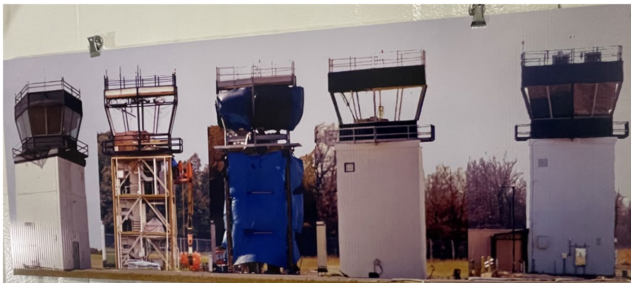
Figure B-14. Phases of 2013-2019 Seismic Retrofit of the PAH ATCT, Courtesy of Barkley Regional Airport
