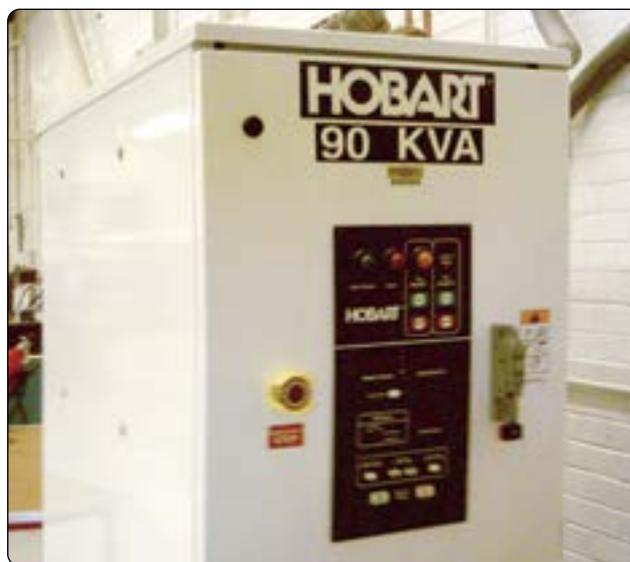
**Figure 1-28.** *A stationary electrical power unit.*
