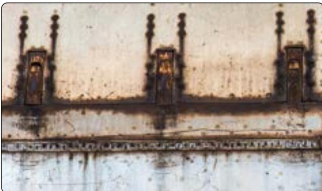
Figure 8-18. Galvanic corrosion.
