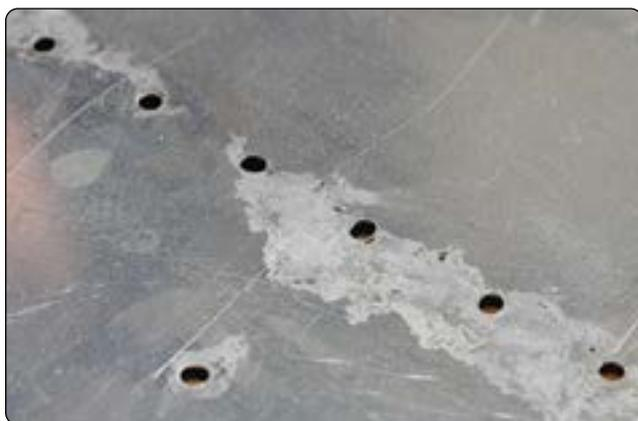
**Figure 8-7.** *Surface corrosion.*
