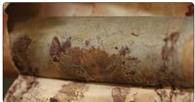
**Figure 8-27.** Rust on structural components.
