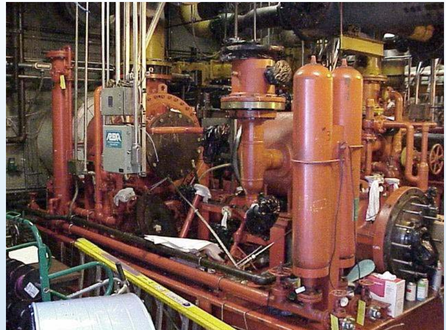
Rotoflow Turbo-expander #3
