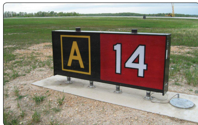
Figure 14-9. Runway holding position sign at takeoff end of Runway 14 with collocated Taxiway Alpha location sign.
