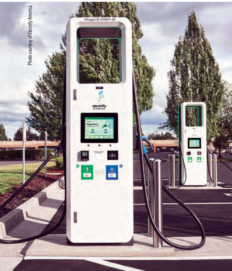
A 350 kW DC Fast Charger. Note the heavy cord and CCS connector.
