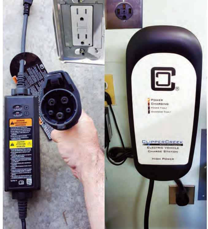
In this photo, we see the difference between Level 1 and Level 2 automotive Electric Vehicle Supply Equipment (EVSE), commonly referred to as chargers, and the different outlets they use.
