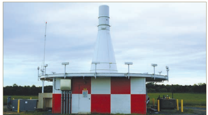
The lower part of VHF airband (108-117.95) is split into 200 narrow-band channels primarily reserved for navigation aids, like this VOR station.
