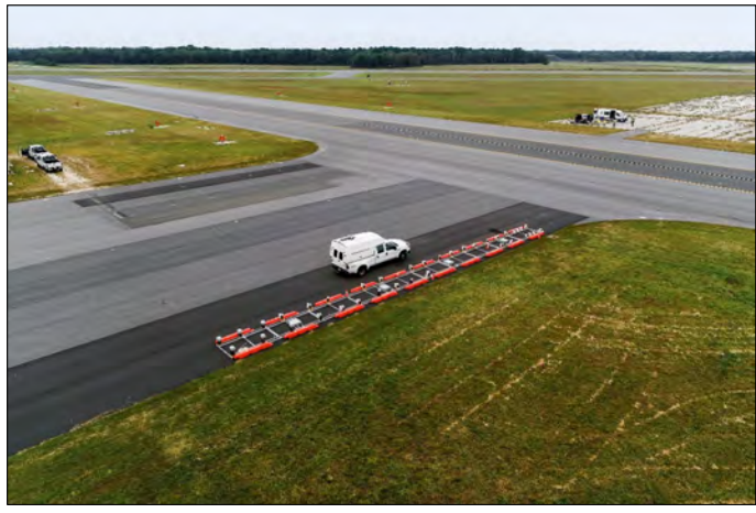
Solar Device Test Beds will have a combined foot print of approximately 100 feet x 70 feet.
