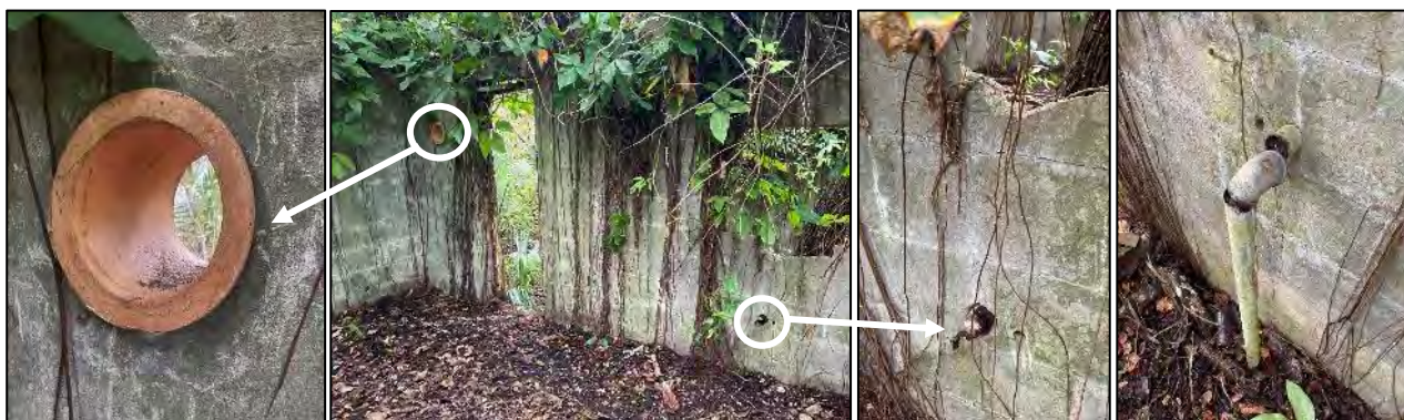
Figure 5.7 Kitchen Area (second photo from left) with a Clay Wall Flue, Thimble for Stove Pipe (left), and Metal Pipe-Interior and Exterior (right).
