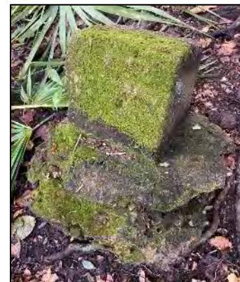
Figure 5.8 Poured Concrete Footer for Porch.
