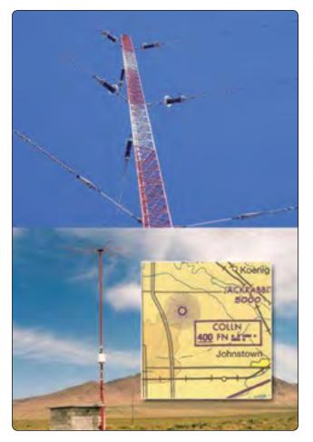
**Figure 11-106.** *Nondirectional broadcast antenna in the LF and medium frequency range are used for ADF navigation.*
