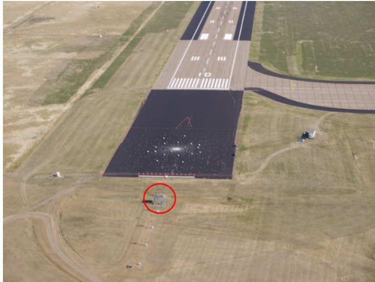
Figure 5-3 - Glasgow runway end with a small structure highlighted by the red circle.
