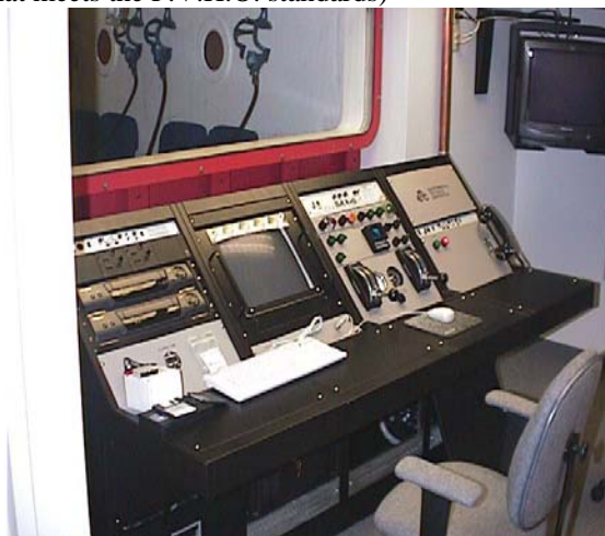
(Control Console with manual and computer controls)
