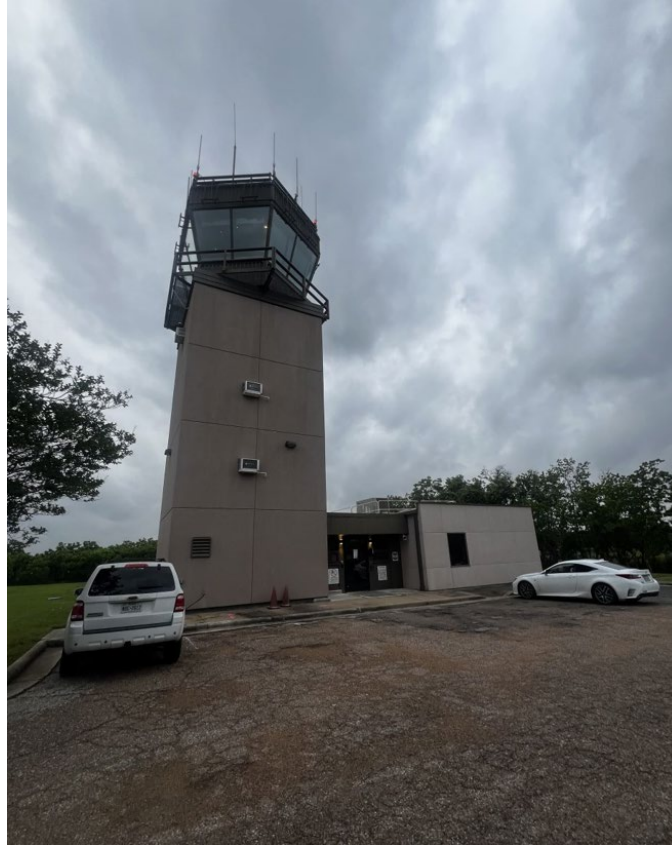
Figure 1-2. Photo of Existing Hunt/AVCO ATCT at DWH
