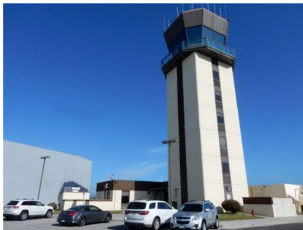
Figure B-8. CMA ATCT (Camarillo, CA) with midsize shaft and regular size 8-sided (chamfered square) Cab, FAA
