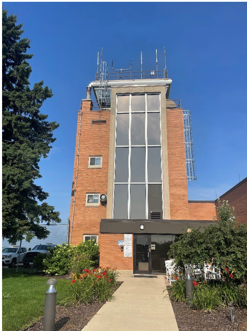
Figure 1-2. Photo of Existing ATCT at RFD
