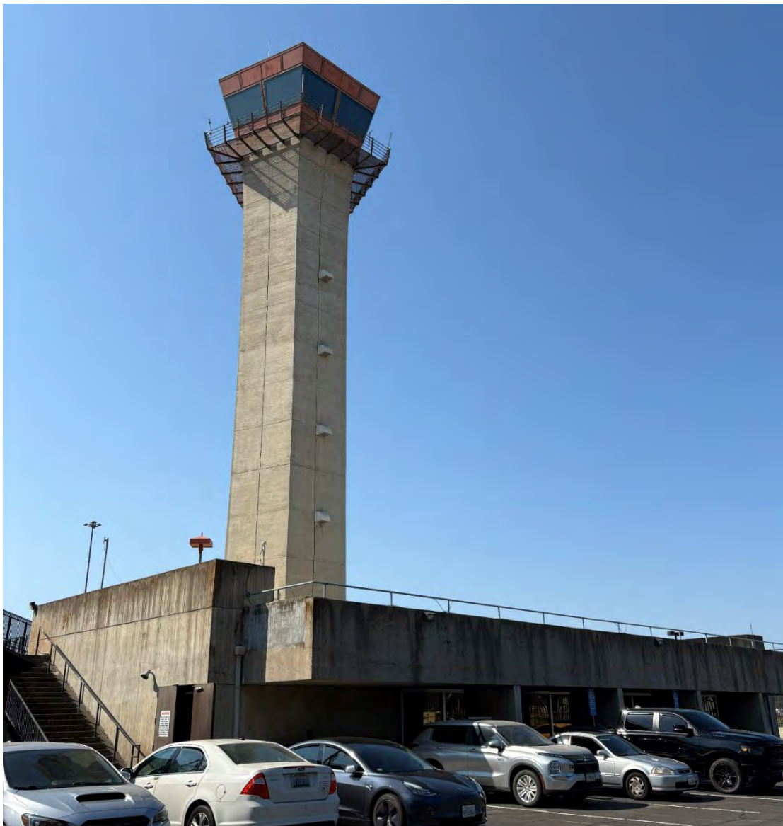
Figure 1-2. Existing SMF ATCT and Base Building
