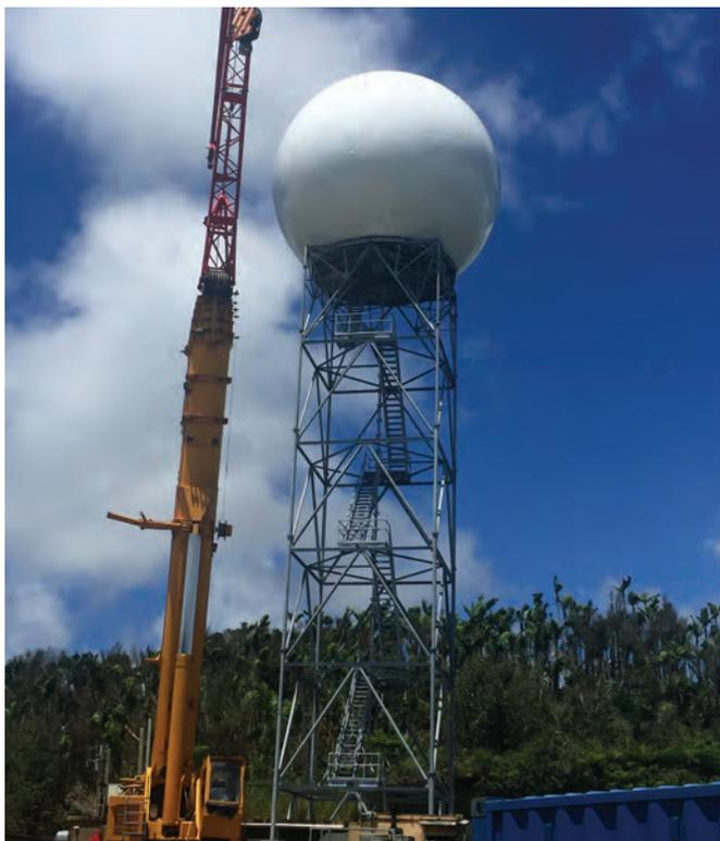
A WSR-88D NEXRAD Doppler weather radar system being repaired after severe storm damage in 2017.
