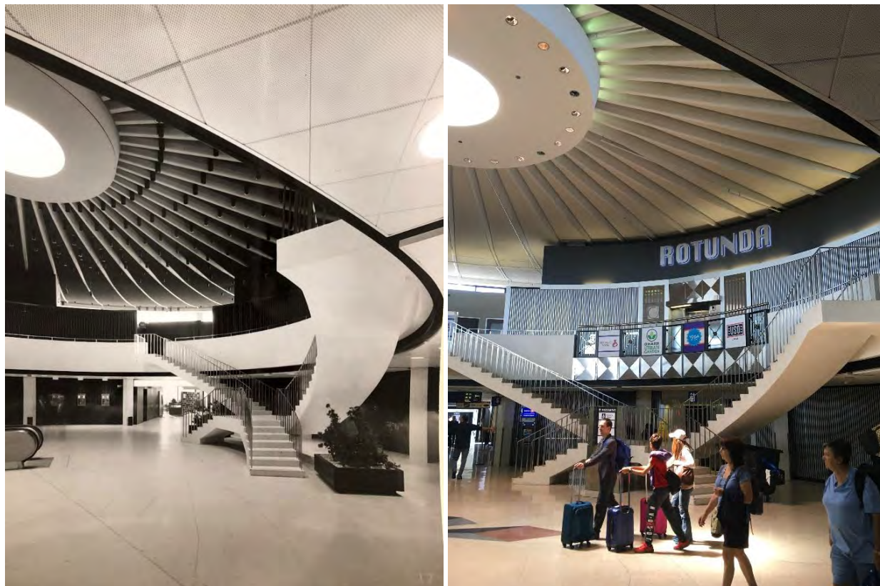
Figure 13 and Figure 14. Historic (left) and current (right) photographs of the Rotunda illustrating changes to the inner atrium at the concourse and mezzanine levels. Changes include removal of original escalator (at far left of Figure 13), installation of decorative terrazzo floor detail, signage added to mezzanine level, installation of non-original ceiling panels, and removal of pendant lights in between ribs. Historic photograph credit: HB-29048, Chicago History Museum, Hedrich-Blessing Collection, © 2019 Chicago Historical Society, all rights reserved.
