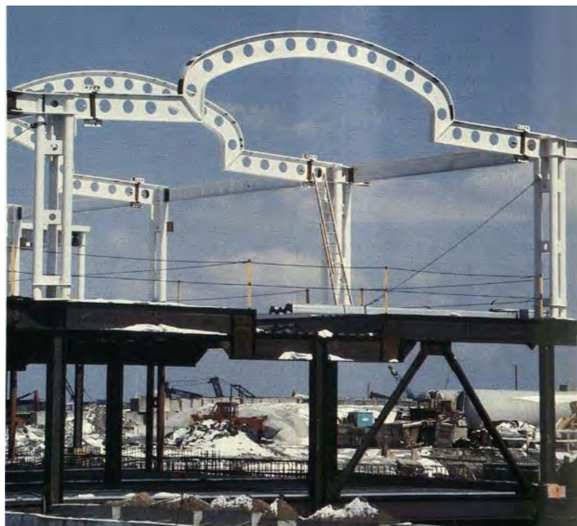
Figure 67. Pre-welded exposed steel structure of Concourse C during construction, 1986. 52
