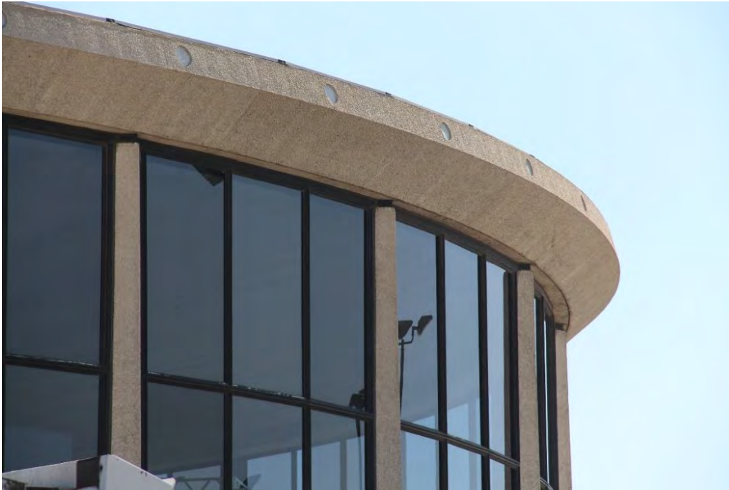
Figure 7. Detail view of sculpted concrete columns that support the concrete perimeter ring at the top of the building. The small circles along the outer edge of the roof are the anchor points for the roof cables.
