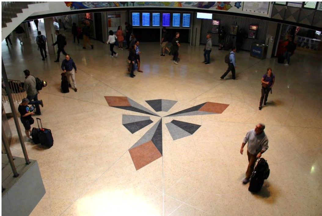
Figure 18. Terrazzo floor with non-original decorative detail located in the inner atrium of the concourse level. The decorative terrazzo floor design was installed after an escalator was removed from this space in the 1990s.
