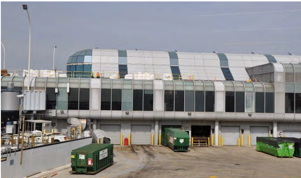
Figure 28. Photograph of work in progress on Concourse B barrel vault and apse, showing the overclad glazing and metal units with clear color variation due to the clean condition of the new materials.
