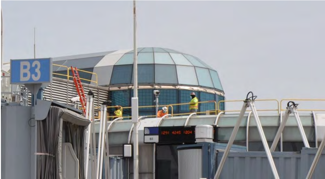
Figure 27. Photograph of work in progress on Concourse B apse showing overclad glazing and metal units on the vaulted area. The butt joints between units are narrower than the original horizontal and vertical dimensions, which are still visible on the vertical end wall.
