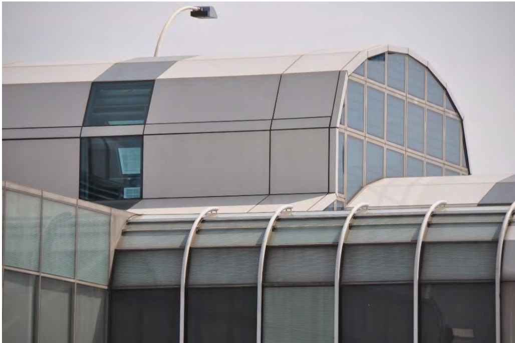
Figure 5. Photograph of Concourse C showing metal panels and glazing over cladding the barrel vault; the butt joints between units are narrower than the original horizontal and vertical dimensions, which are still visible on the vertical end wall.
