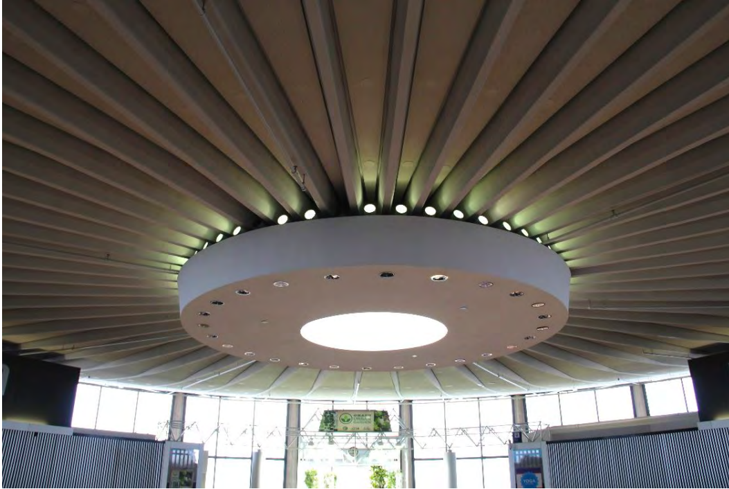
Figure 11. Oculus and axial ribs at the center of the Rotunda provide a focal point for the space. Recessed lighting at the oculus is not original.
