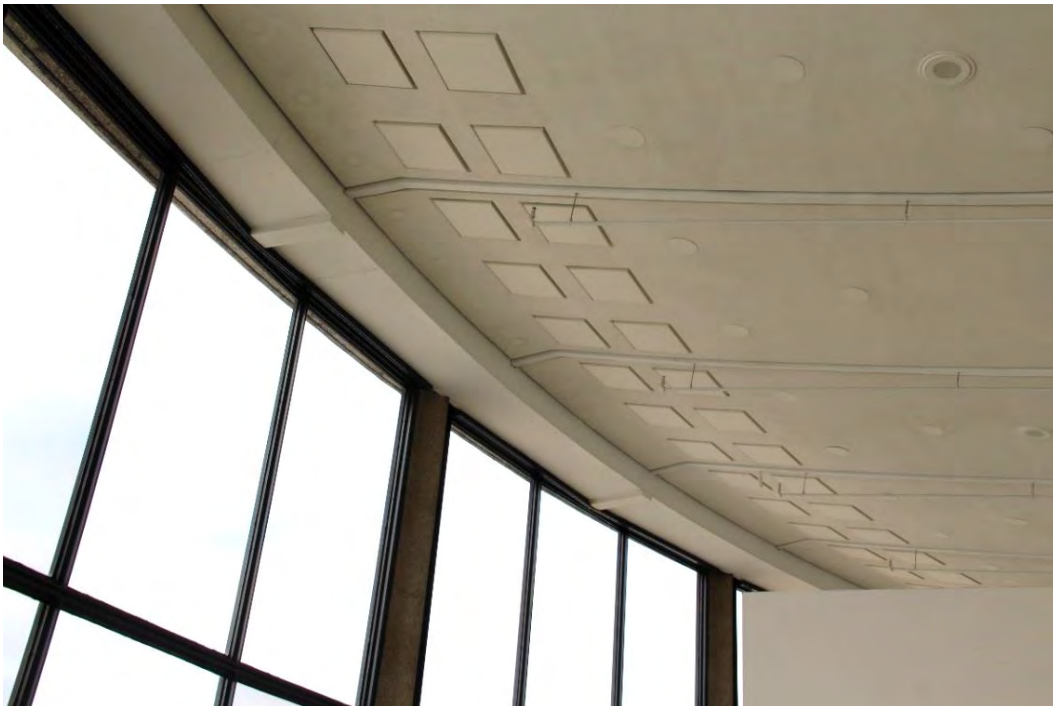
Figure 12. Parallel rows of square panels extend around the outer edge of the ceiling. Note circular infilled areas where original ceiling mounted lighting was removed.
