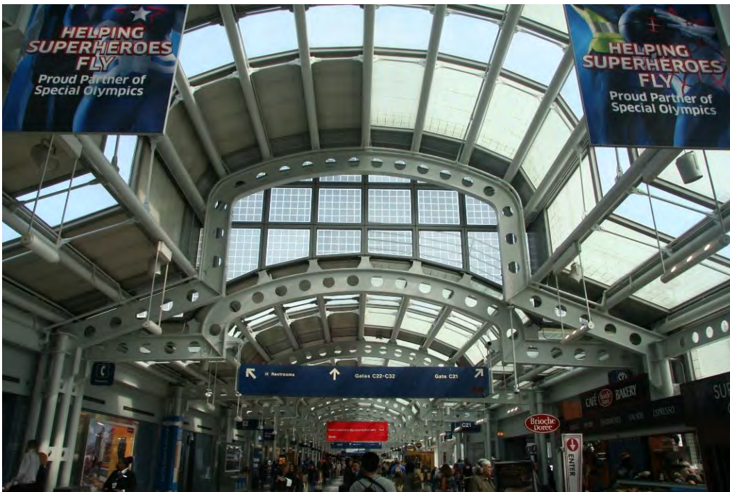
Figure 18. April 2019 photograph of the interior of Concourse C, showing barrel vault along main circulation spine before roof repair project.
