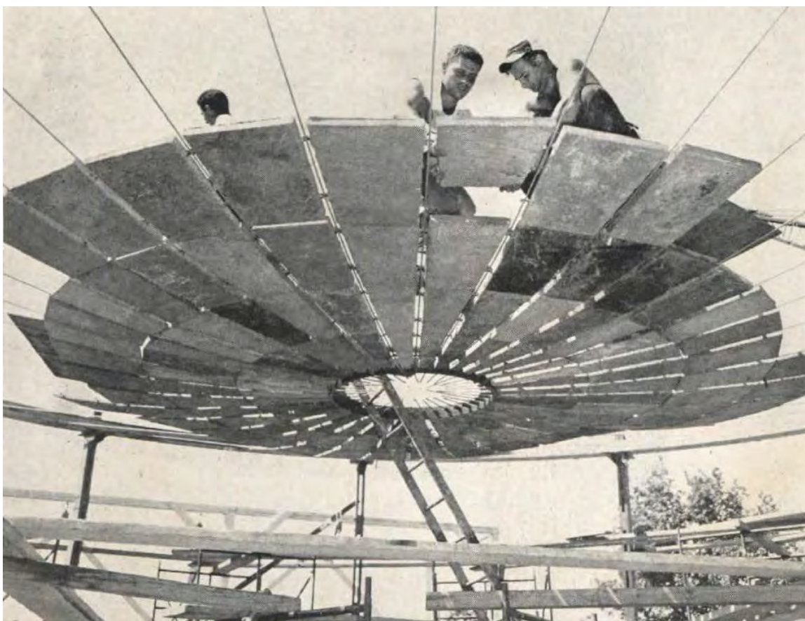
Figure 46. Radial cable-suspended roof under construction at Camp Columbia in 1956. 93
