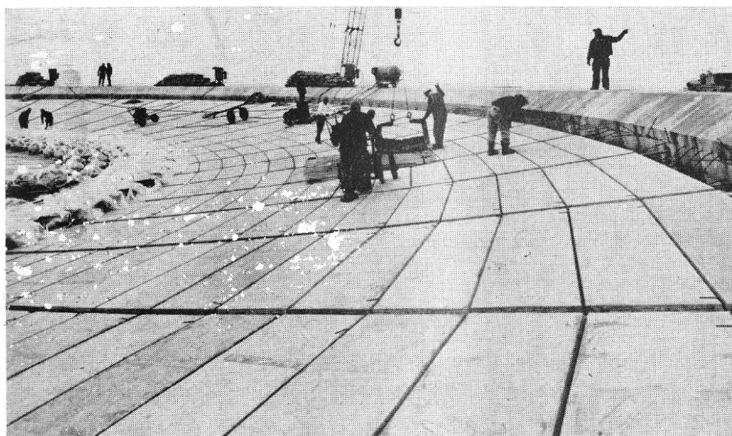
Figure 38. Photograph of the cable-suspended roof under construction in 1962. 39
