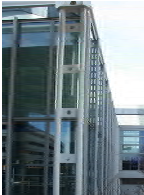
Figure 13. Curtain wall structure.
