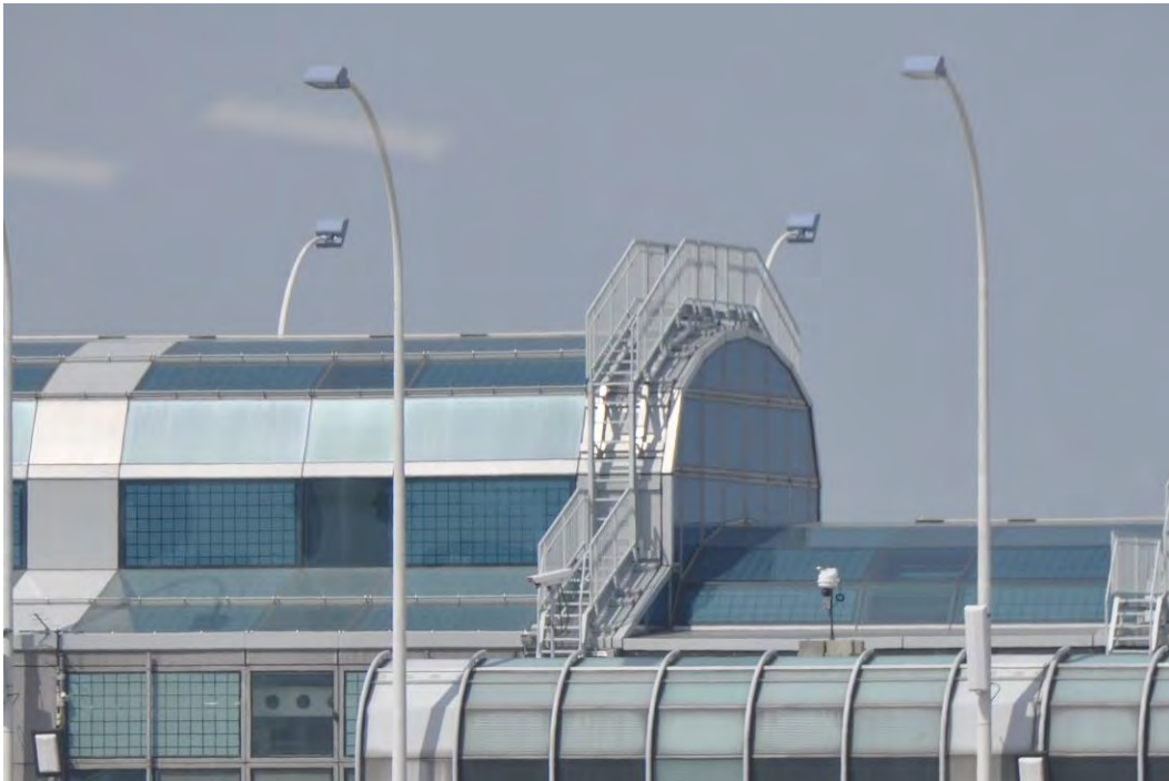
Figure 14. Photograph of the exterior of Concourse C after completed work, showing new roof elements for access and ice/snow mitigation.
