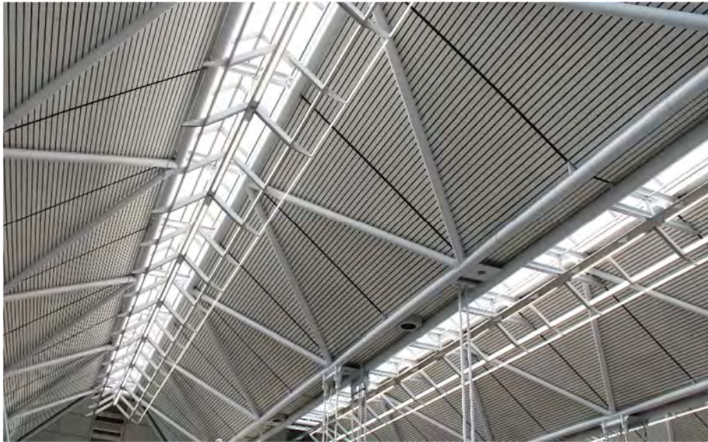
Figure 20. Folded plate ceiling and bladed light fixtures.
