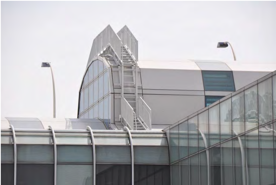
Figure 16. Photograph of the exterior of Concourse C after completed work, showing detail of new metal stairs and overclad panels and glazing units.
