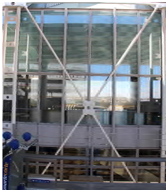
Figure 10. Ticketing exterior wall X-brace and curtain wall division.
