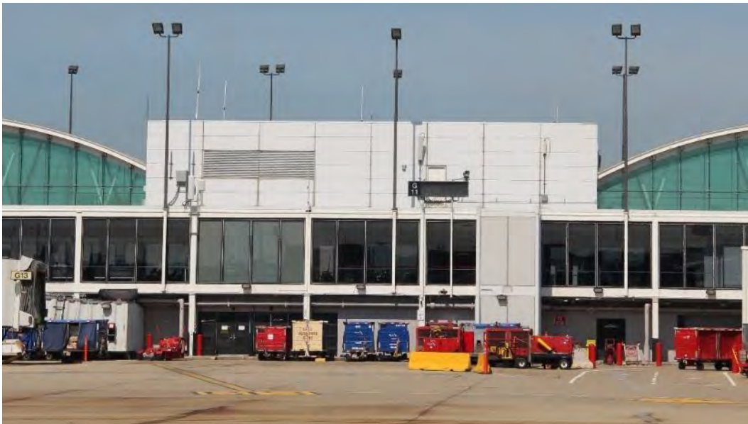
Exterior of Concourse G, showing window grid-block pattern at the first level and penthouse clad in phenolic wall panels.
