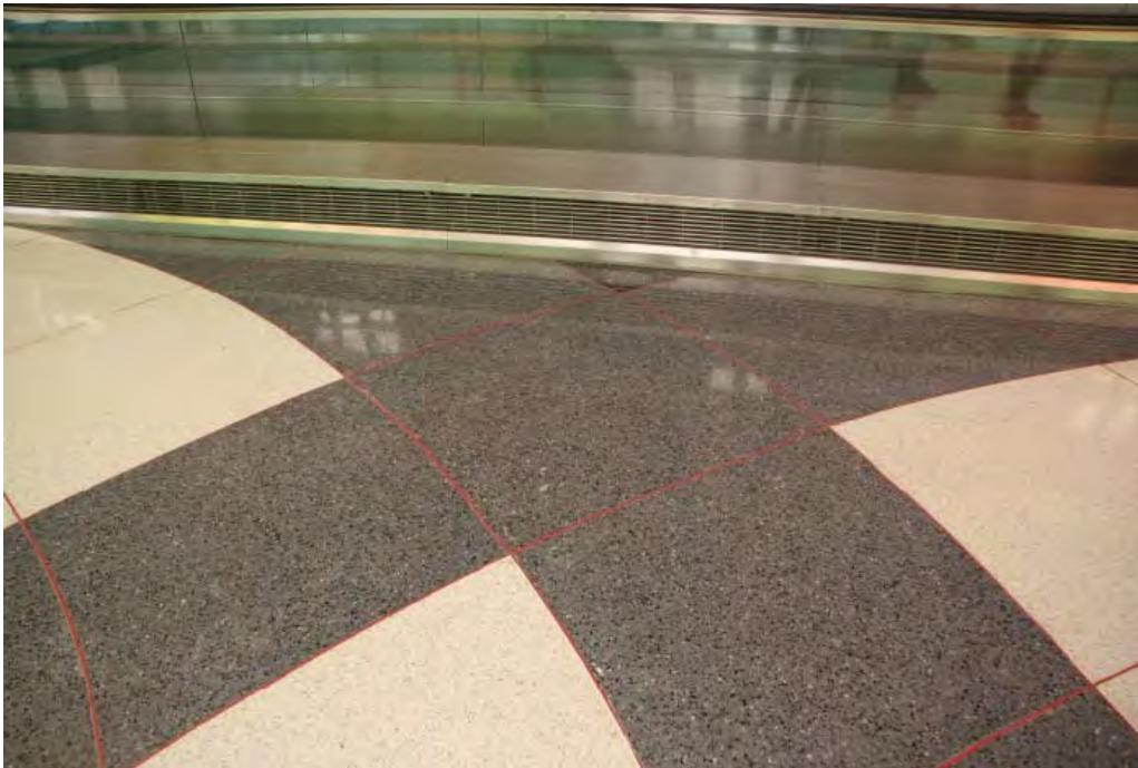
Figure 60. Detail of terrazzo flooring.
