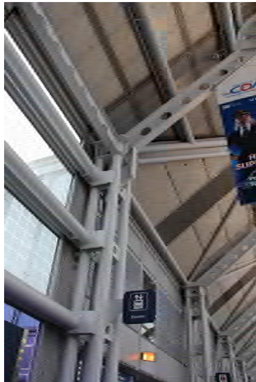
Figure 38. Concourse girder, beam, and column connection point.
