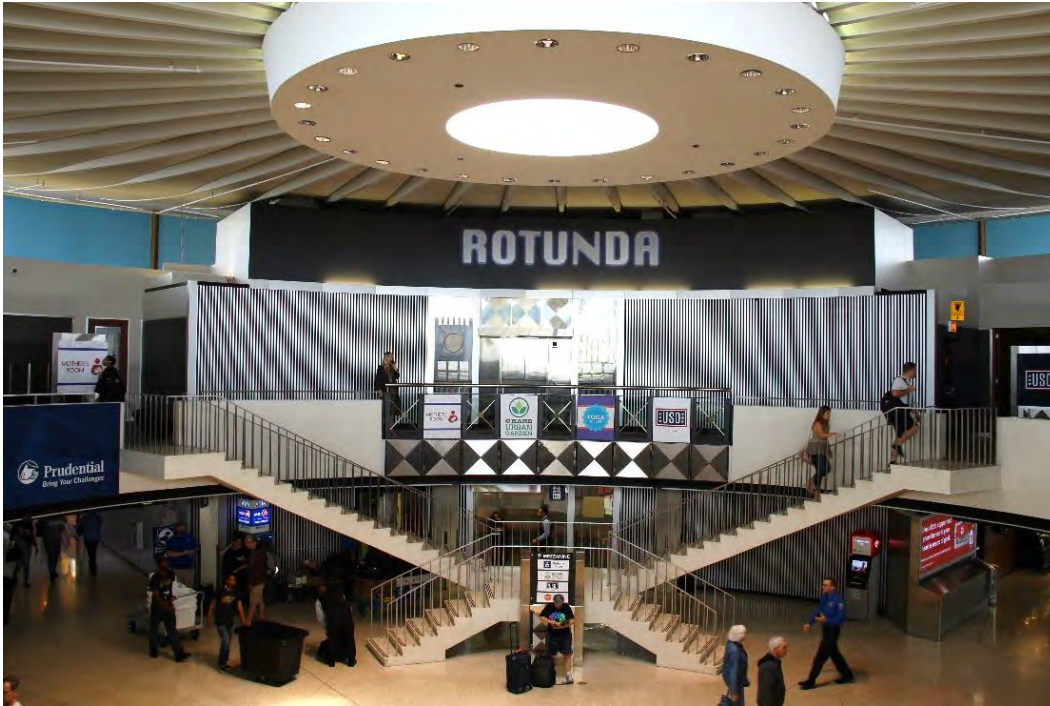
Figure 15. Overview of the inner atrium and concrete staircases. Modern signage has been added at the mezzanine level, as well as slatted metal covering over original wood ribbing.
