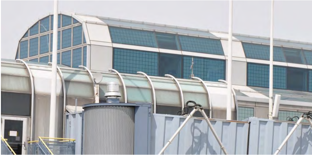
Figure 3. Photograph of the barrel vault along the spine of Concourse C.
