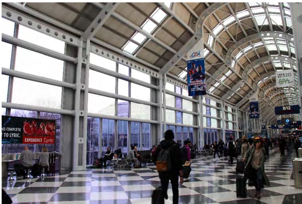
Figure 39. Concourse B curtain wall glazing.
