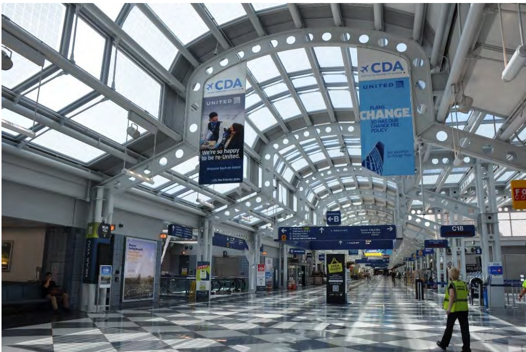
Figure 20. Photograph of the interior of Concourse C after completed work, showing barrel vault along main circulation spine with new glazing units throughout. It is not discernible that units are on now on outside rather than inset into framing.
