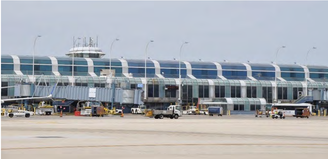
Figure 15. Photograph of the exterior of Concourse C after completed work, showing overall effect of the overcladding including color variation.
