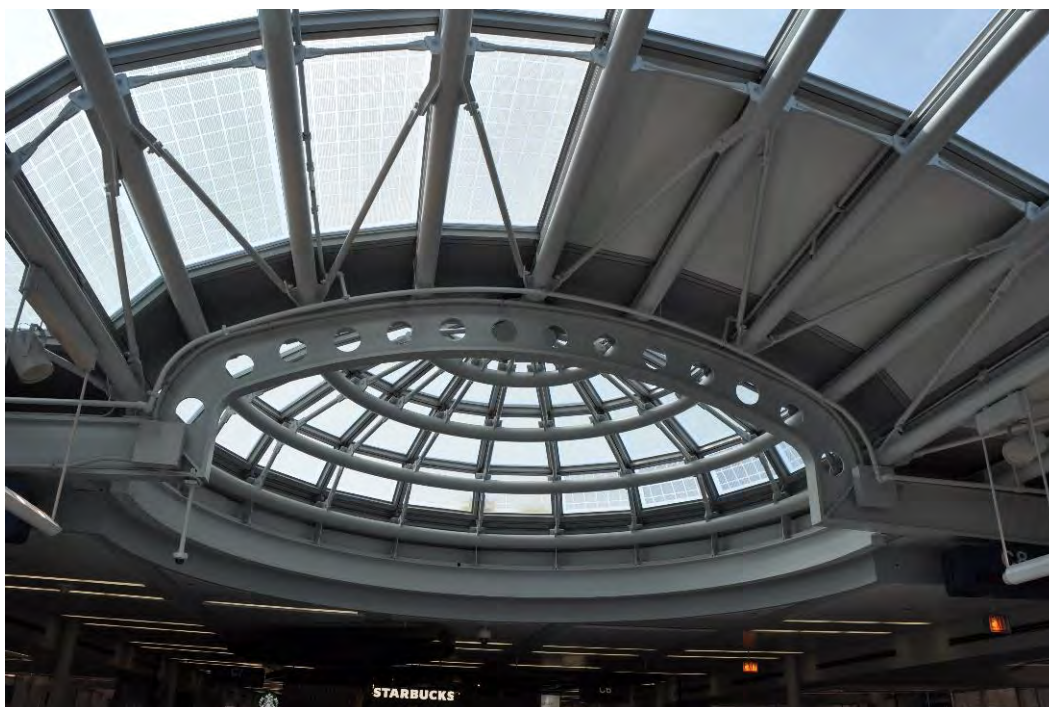
Figure 23. Photograph of the interior of Concourse C after completed work, showing apse at end of main circulation spine. The border around frit block pattern and variation in hue can be discerned by a trained eye.
