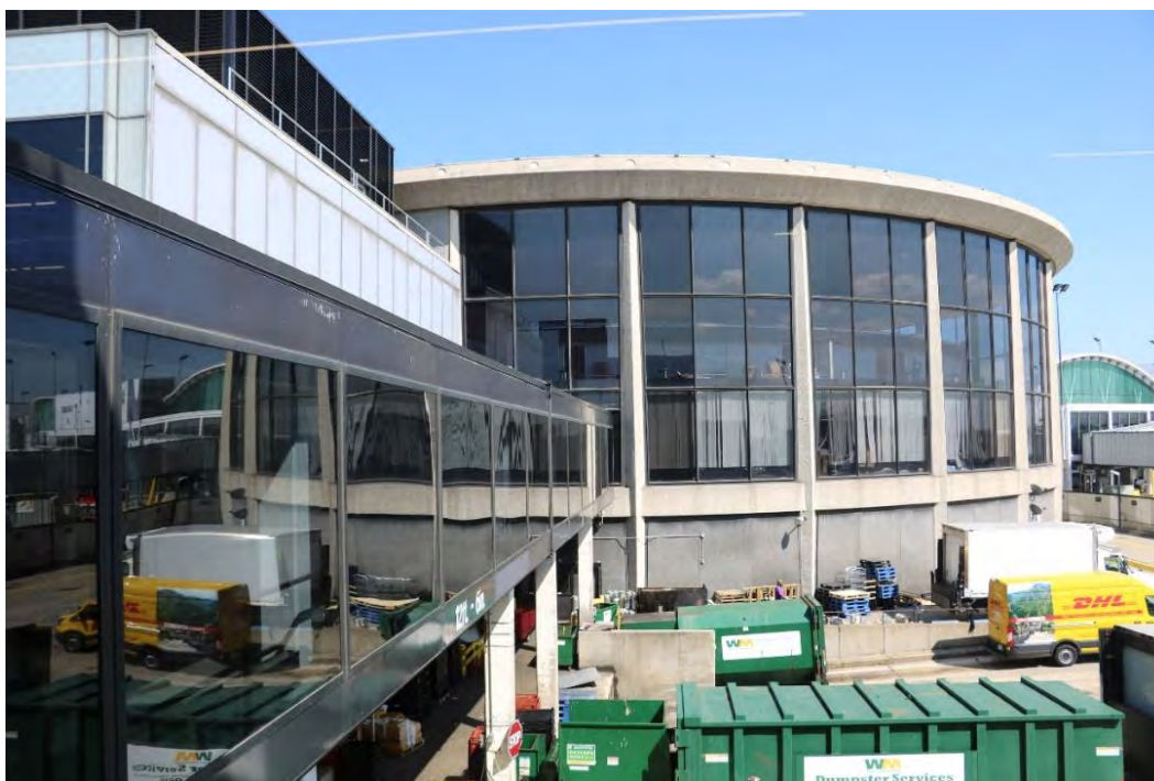
Figure 6. Overview of Rotunda exterior, illustrating the sculpted concrete columns, glass curtain walls, and concrete perimeter ring. A service entrance at the apron level is located directly below the enclosed glass walkway near the center of the photograph.
