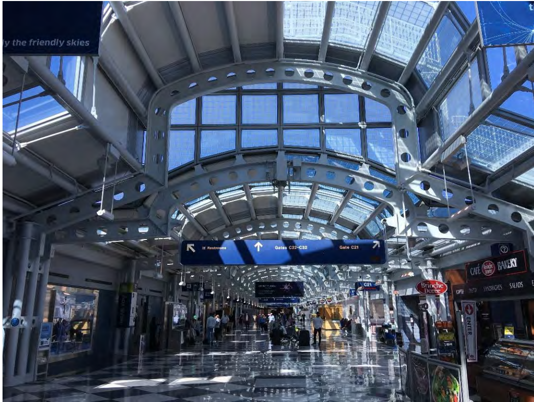
Figure 21. Photograph of the interior of Concourse C after completed work, showing the main circulation spine. The subtle differences of tinted glass and border around the frit pattern can be discerned by a trained eye.
