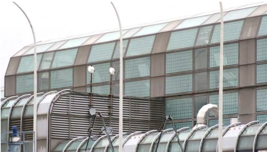
Figure 5. Curtain wall enclosure with exterior aluminum arched structure shown in forefront.
