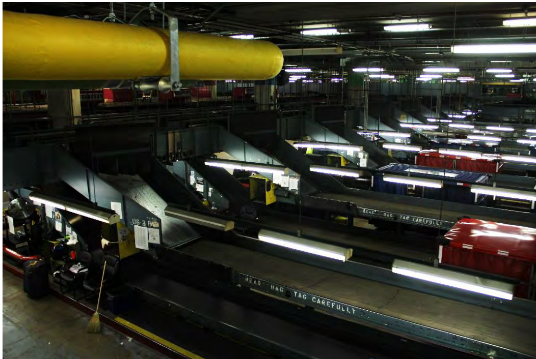
Figure 64. Rows of conveyor belts and metal chutes at the baggage handling area at the tunnel level. Carts can be seen in some aisles.
