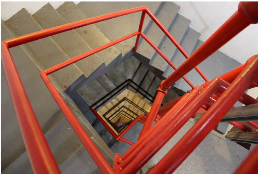
Figure 24. Detail of shaft square spiral staircase and painted iron stair rail.
