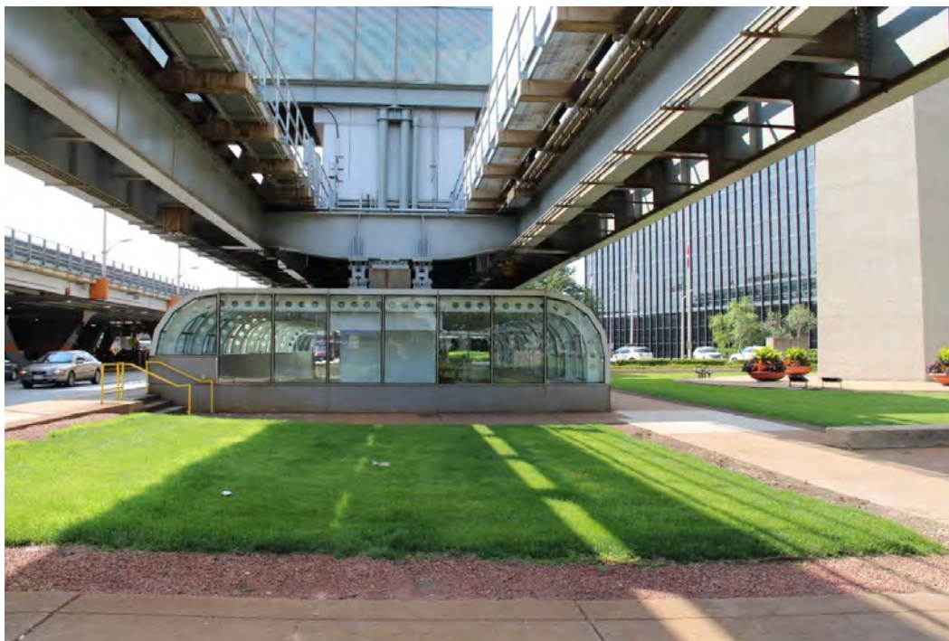
Figure 15. Southeast facade of atrium enclosure showing steel trusses with punched holes through the webs.
