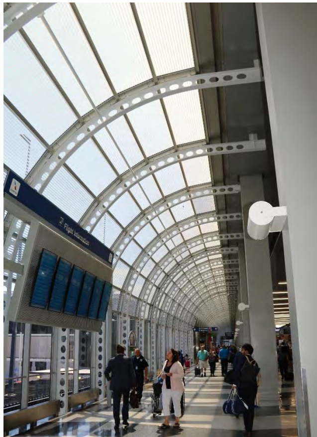
Figure 27. Detail of the exposed, interior, steel, semi-arch structure of the south elevation addition to the main terminal building.
