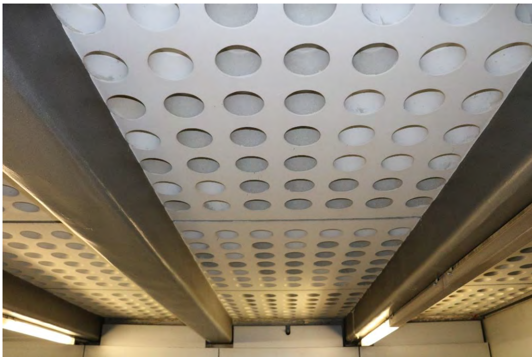
Figure 41. Detail of the dimpled concrete ceiling above the mid-landing of the stairs that lead from the apron-level baggage claim to the pedestrian concourses toward the parking garage and CTA station.
