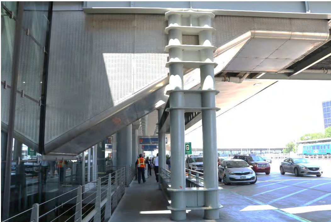
Figure 15. Steel supports at the elevated bridge from the main terminal building to the ATS.
