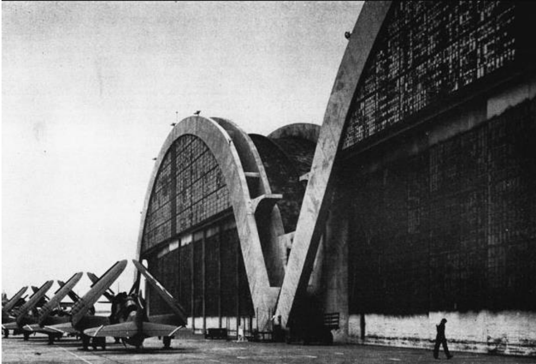
Figure 91. Concrete arch hangars at the San Diego Naval Air Station. 81
