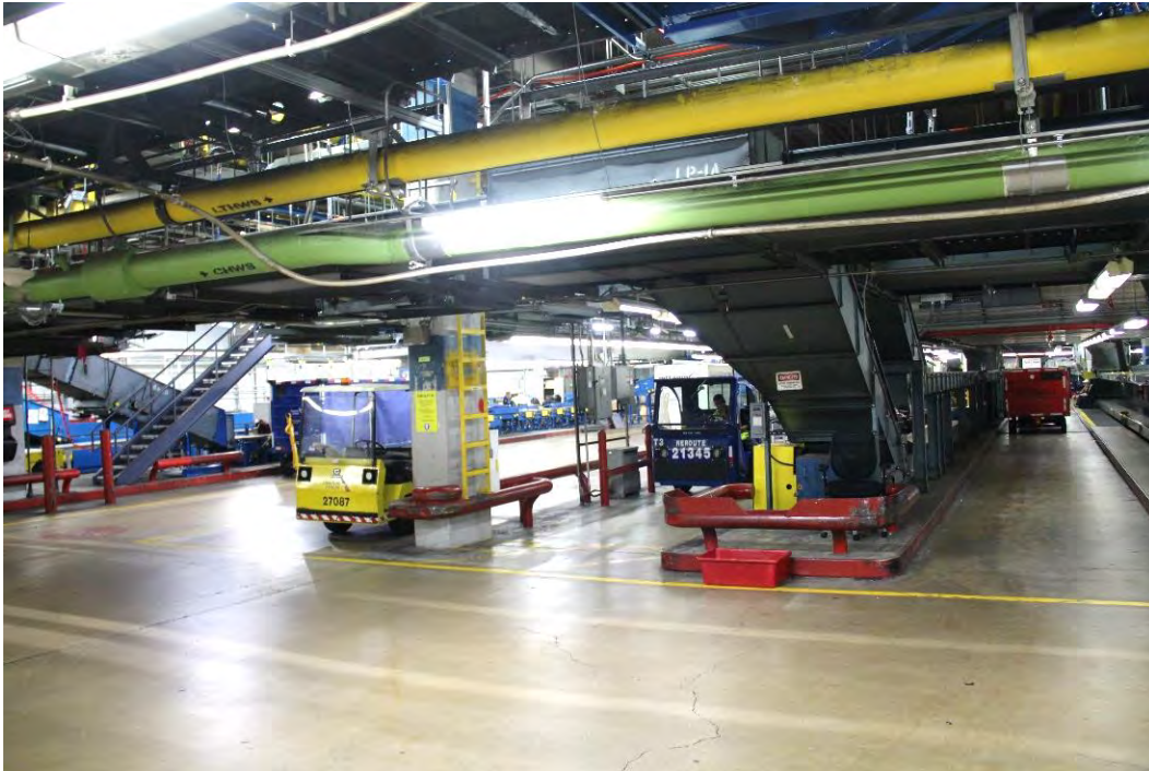
Figure 65. Aisles between rows of conveyor belts and metal chutes at the baggage handling area at the tunnel level.
