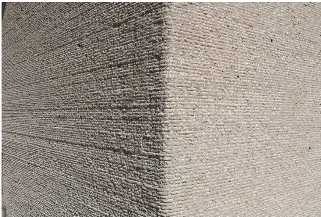
Figure 7. Detail of horizontally grooved, bush-hammered finish on tower shaft.
