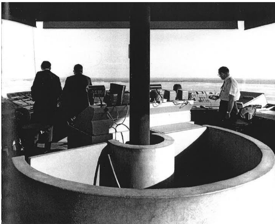
Figure 46. View of standardized cab interior showing equipment consoles. 77
