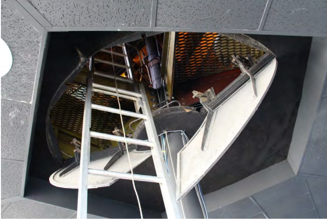
Figure 27. Opened hatch to roof showing extension ladder access.
