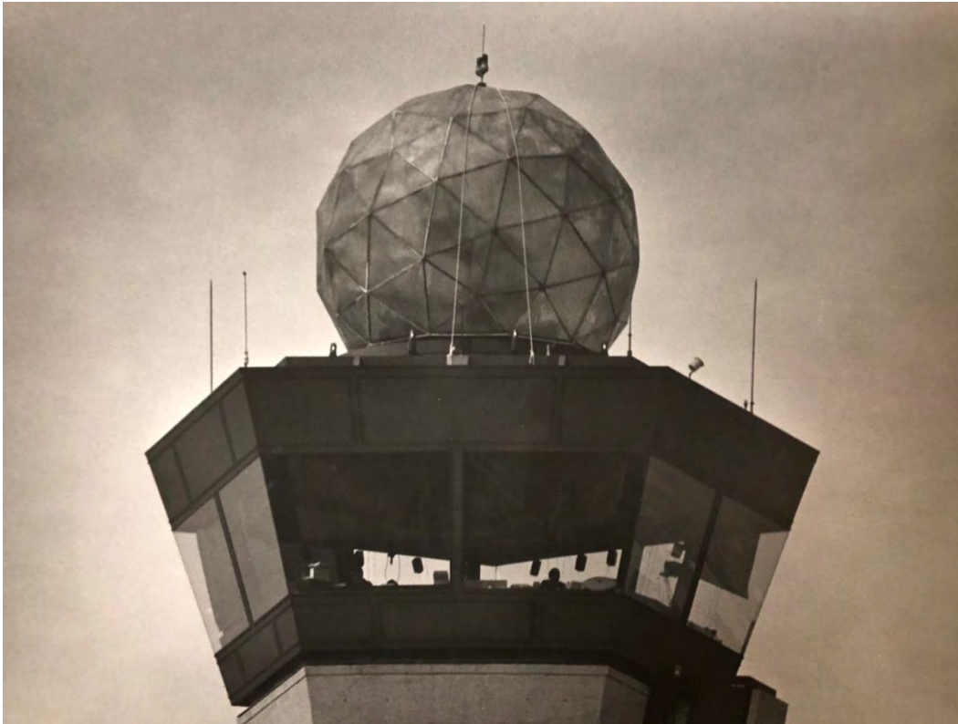
Figure 16. Image of tower cab showing radome and a portion of the window washing bucket to the right. Historic photograph credit: ICHI-176501, Chicago History Museum, John McCarthy, photographer, © 2019 Chicago Historical Society, all rights reserved.
