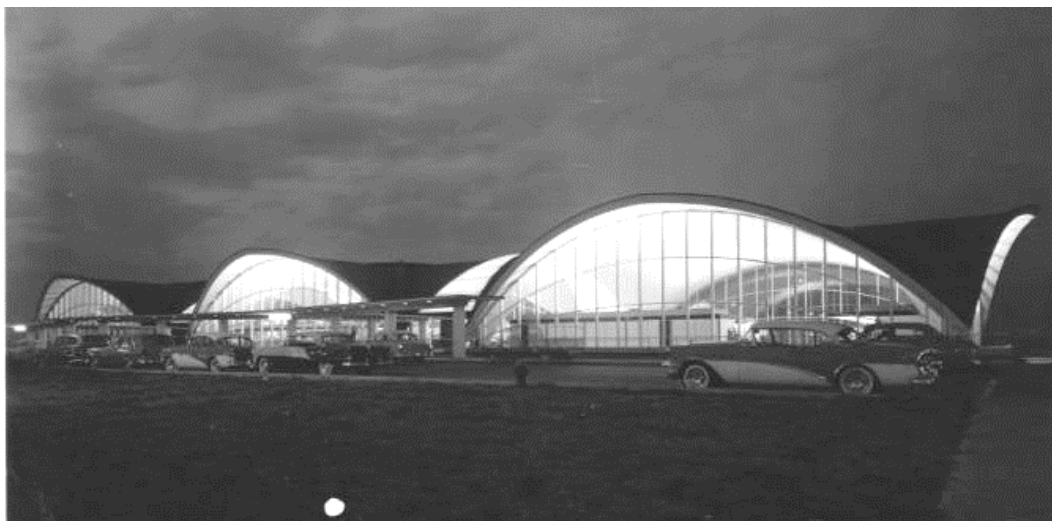
Figure 92. Concrete arches of the terminal at Lambert International Airport. 82
