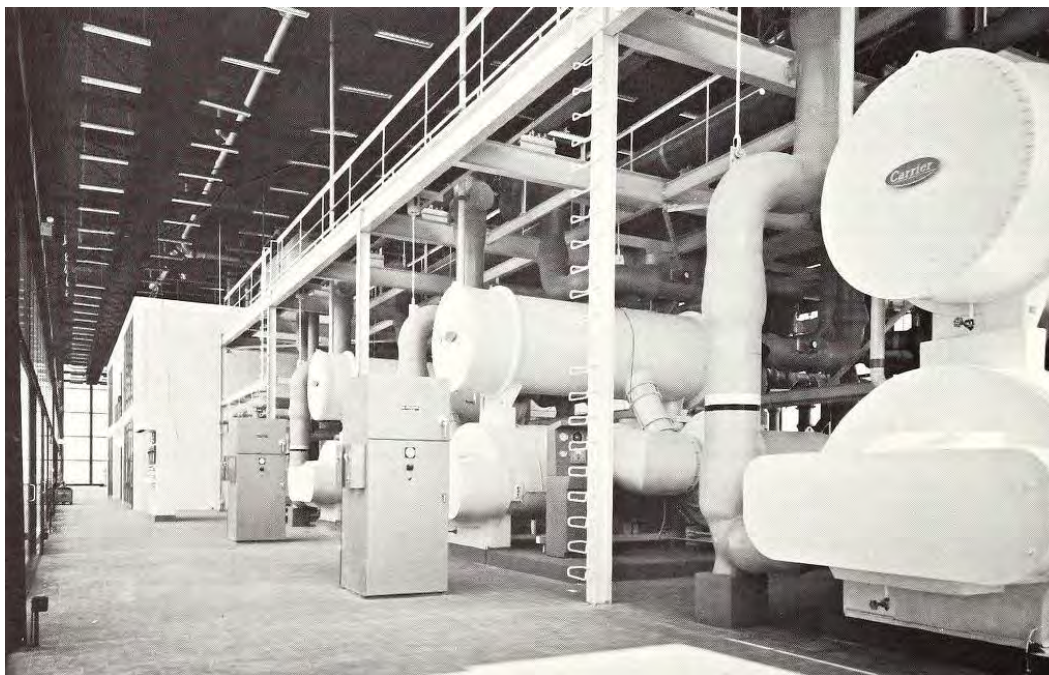
Figure 67. Interior view of the H&R Building showing three Carrier hermetic centrifugal chillers painted white, 1962. 86
