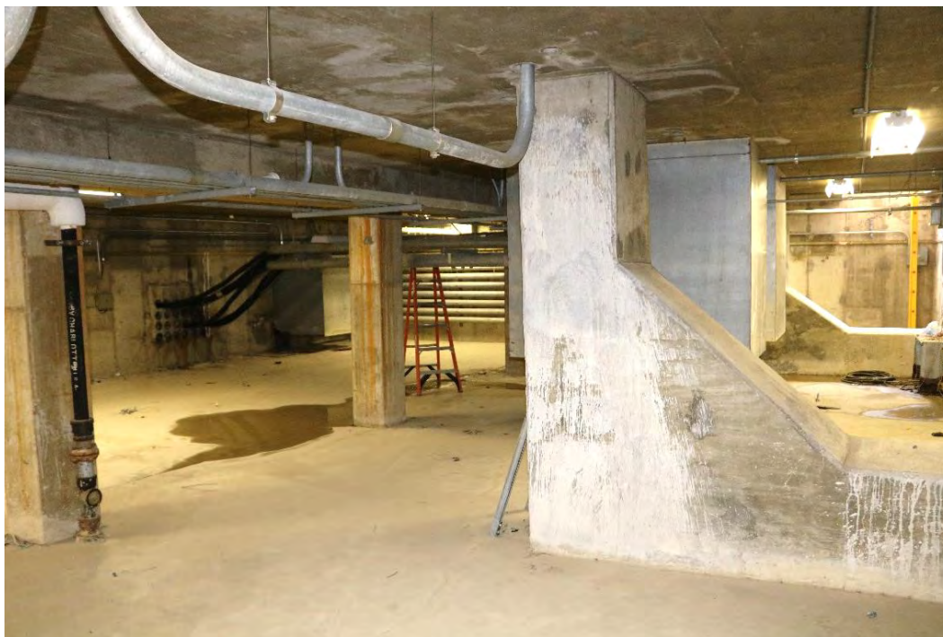
Figure 44. Basement level of the City Substation, with concrete-encased conduit visible at right.
