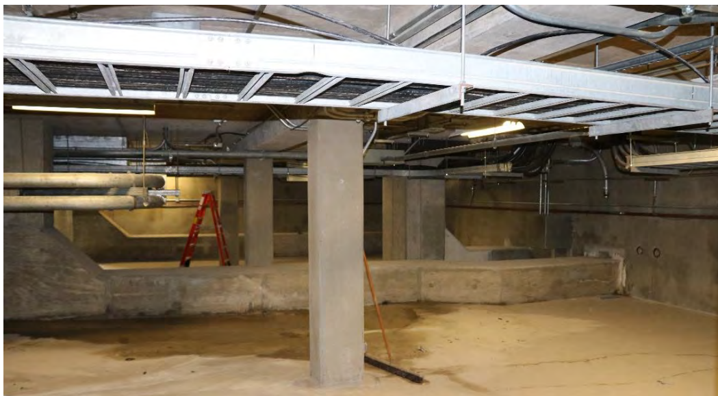
Figure 49. Basement of the RB 40 Substation, with concrete-encased conduit shown entering the building at center and background.
