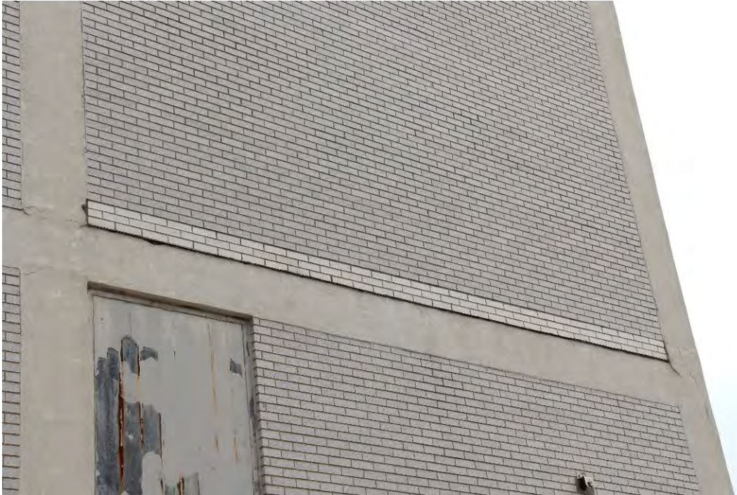
Figure 8. Detail of areas at the south and east elevations that exhibit courses of replacement exterior bricks, view facing northeast.
