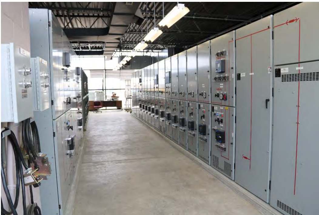
Figure 48. Switchgear and switchboards on the interior of the RB 40 Substation.
