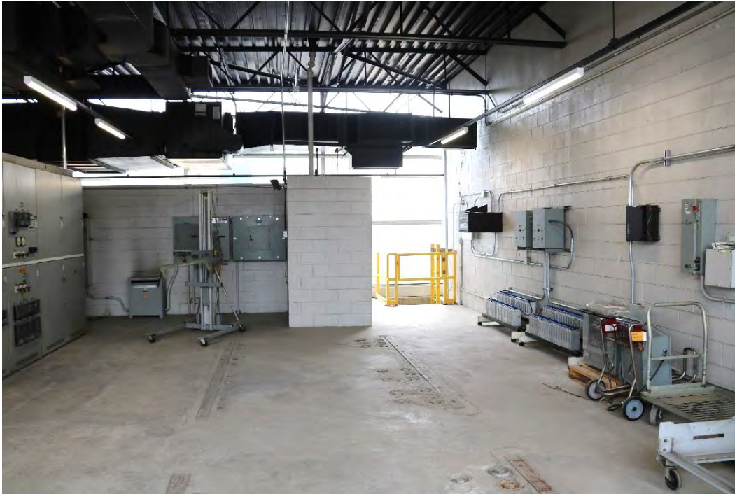
Figure 42. Interior of the City Substation. Switchgear equipment is visible at left, the free-standing concrete-block wall is visible at center, and an access ladder for the basement is visible in the background.
