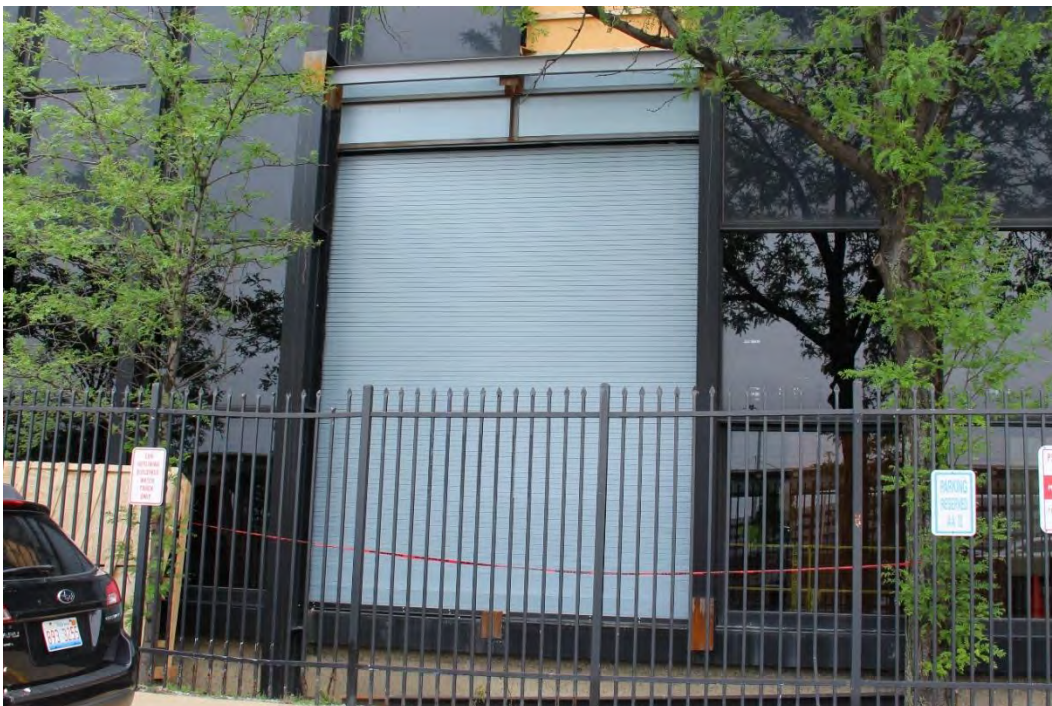
Figure 9. Temporary metal overhead sliding doors on west elevation to facilitate replacement of high-temperature water generators within the building.
