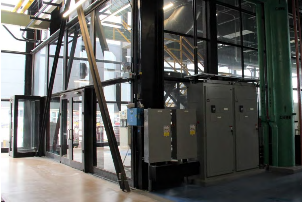
Figure 18. Electrical vault at the southwest corner showing window wall enclosure and both entries from the north-south access aisle.
