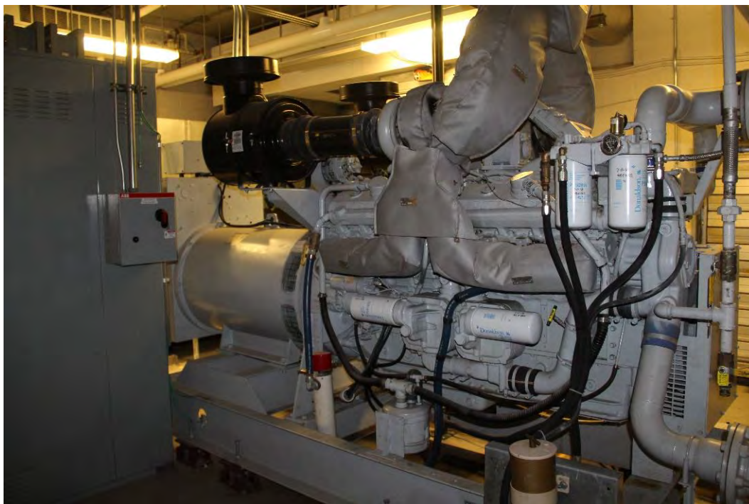
Figure 24. Diesel generator in the basement level.
