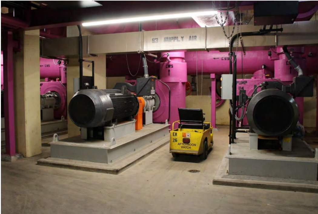
Figure 34. Several condensers are integrated into the refrigeration system, processing water from ancillary cooling towers and delivering it to chillers on the ground level.
