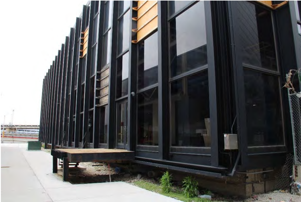
Figure 8. Elevated platform at a secondary entrance, temporary plywood for window replacements, and building overhanging the foundation on the south elevation, view looking west.
