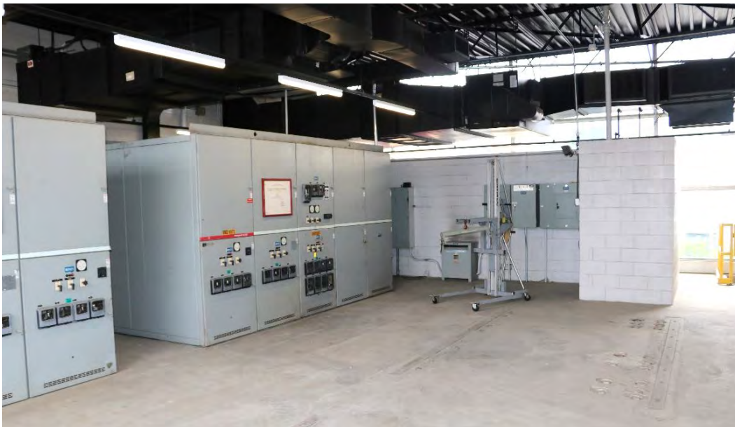
Figure 43. Switchgear equipment on first floor of the City Substation.
