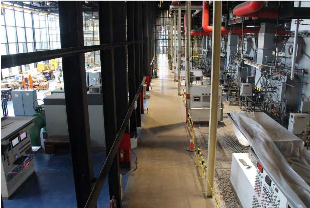
Figure 16. North-south access aisle showing original H-shaped columns and four high-temperature water generators to the right, view from the second mezzanine level (described below).
