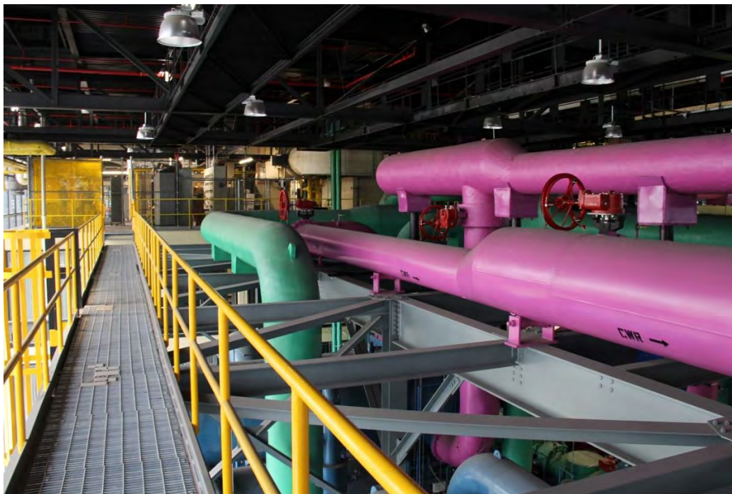
Figure 30. View from a second-mezzanine-level catwalk showing the secondary structural system supporting piping, platforms, and catwalks, and industrial pendant-hung high-bay lighting.
