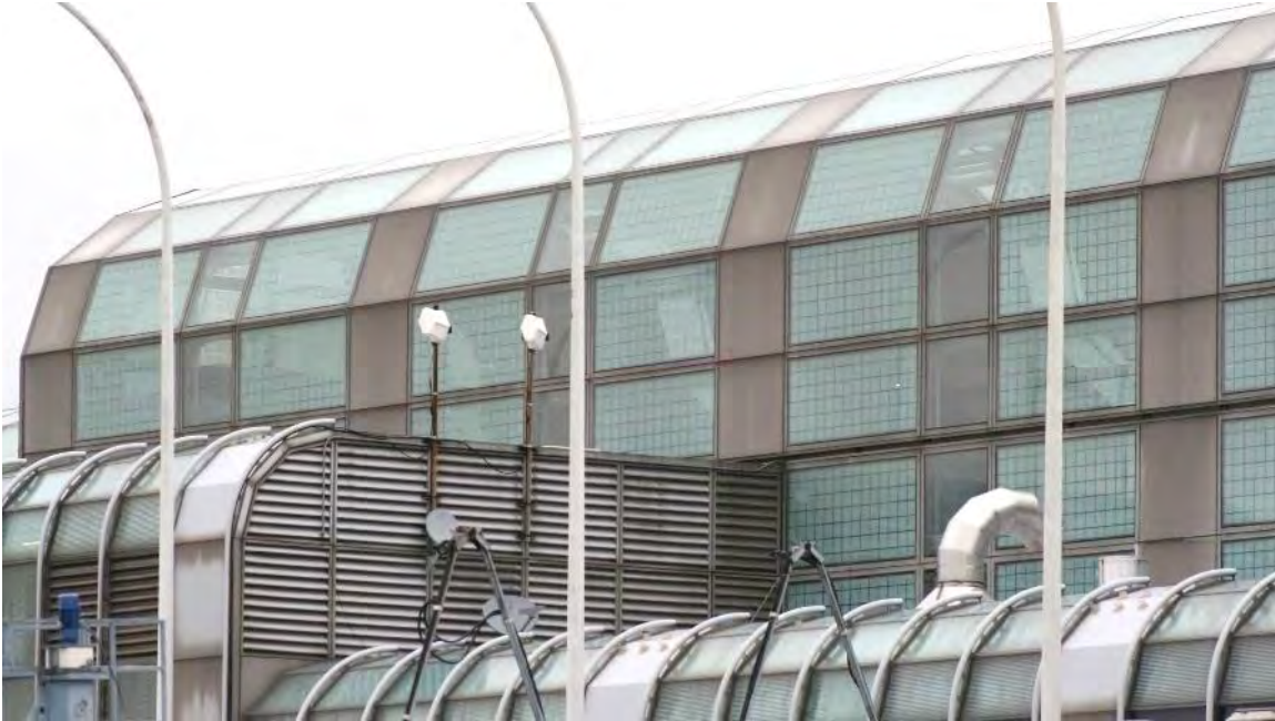
Curtain wall enclosure with exterior aluminum arched structure shown in forefront.
