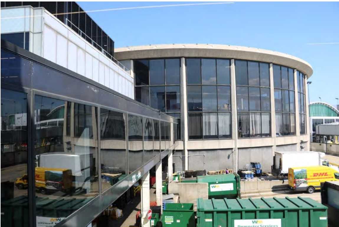
Overview of Rotunda exterior, illustrating the sculpted concrete columns, glass curtain walls, and concrete perimeter ring. A service entrance at the apron level is located directly below the enclosed glass walkway near the center of the photograph.
