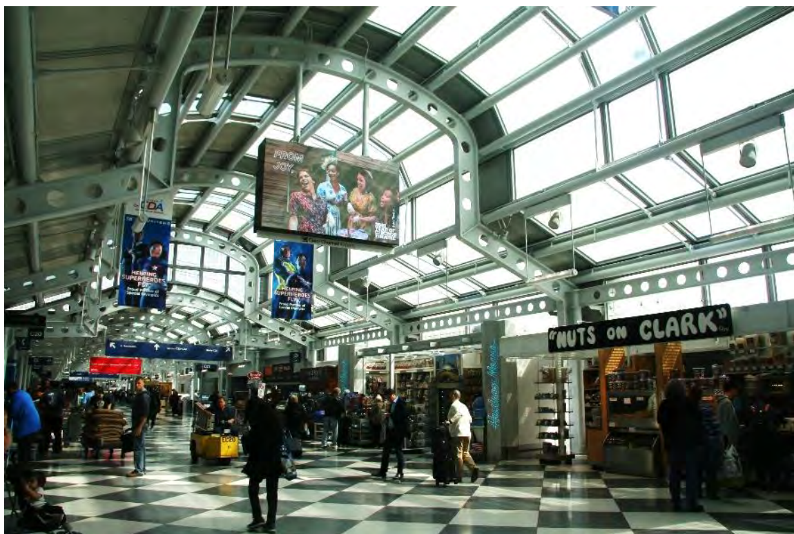
Figure 46. Character-defining features of Terminal 1 including its expansive and integrated vaulted glass curtain wall spaces, along with the stylistic exhibition of the structural engineering seen in the detailed exposed steel structural system with circular cutouts in the webs of beams and girders, primarily visible on the interior of the building.
