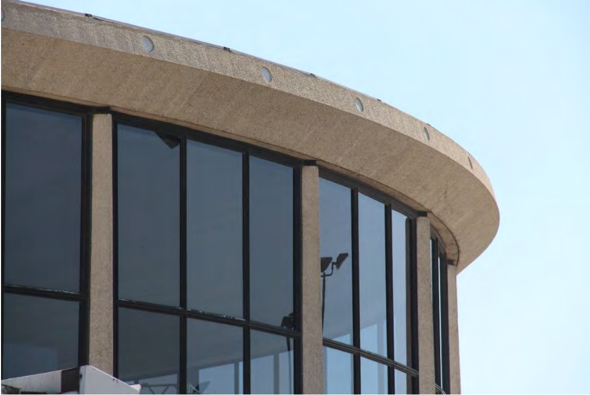
Detail view of sculpted concrete columns that support the concrete perimeter ring at the top of the building. The small circles along the outer edge of the roof are the anchor points for the roof cables.
