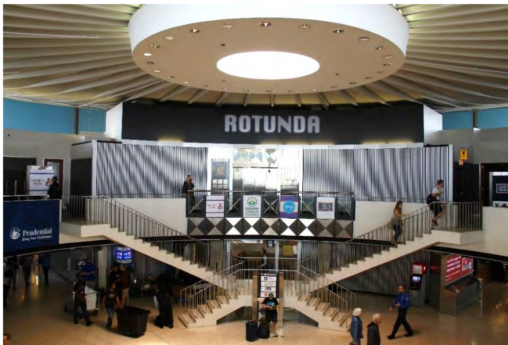
Figure 48. Character-defining features of the Rotunda including double-height interior atrium space and radial cable-suspended roof system resulting in column-less interior space.
