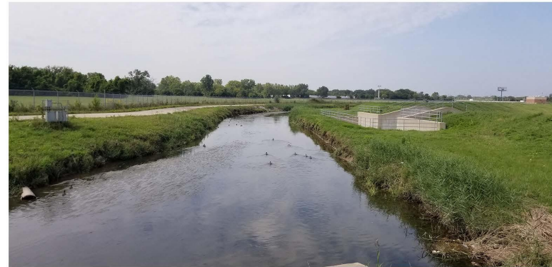
Photo 120. Higgins Creek - Section 1, General site, View to the north
