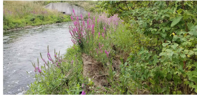
Photo 126. Higgins Creek - Section 3, Higgins creek wracking
