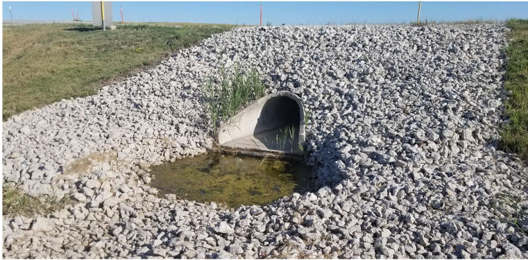
Photo 149. NE19-021, General site, culvert. View to the north
