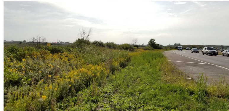
Photo 92. Ditch 32, General site, View to the west
