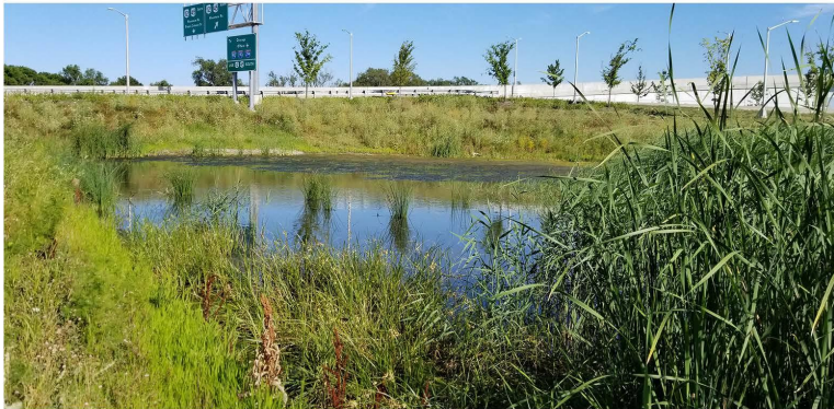
Photo 155. NE19-023, General site, View to the south
