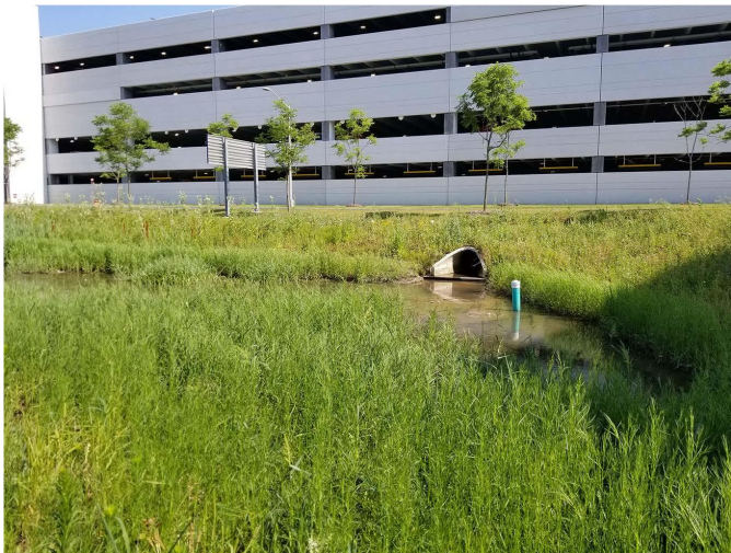
Photo 135. NE19-015, General site, View to the south
