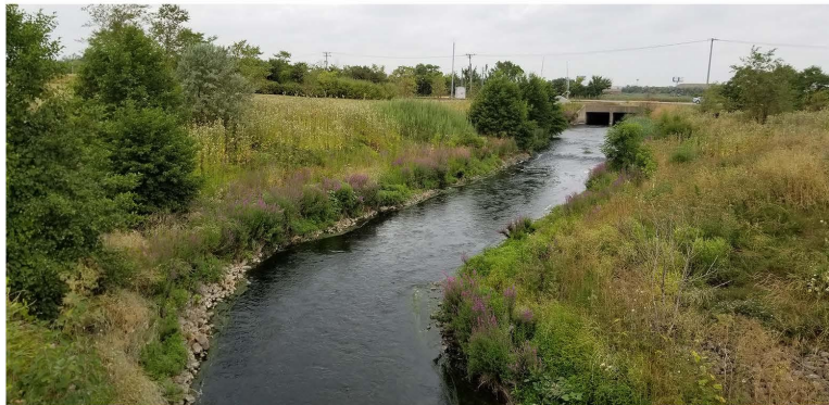
Photo 123. Higgins Creek - Section 3, General site, View to the north
