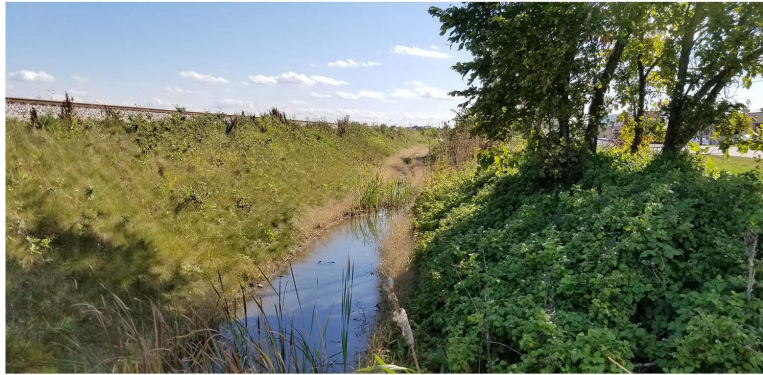
Photo 81. Ditch 25, General site, View to the south
