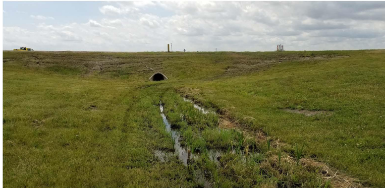
Photo 141. NE19-019, General site, culvert entrance. View to the south
