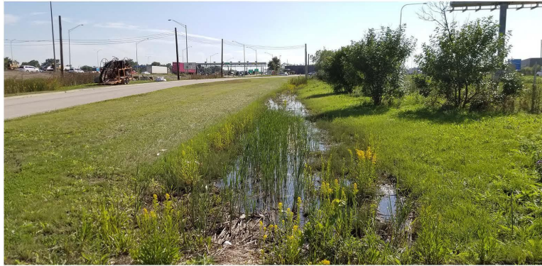
Photo 85. Ditch 28, General site, View to the west
