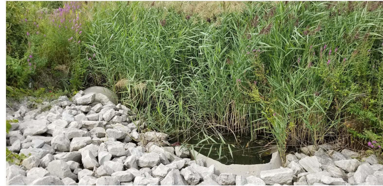
Photo 102. Ditch 39, East culverts, View to the west
