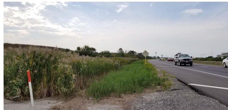
Photo 112. Ditch 44, General site, View to the west
