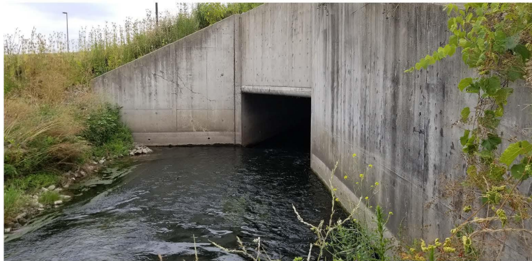
Photo 127. Higgins Creek - Section 3, South culvert. View to the south
