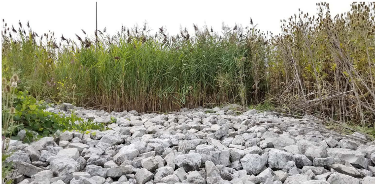
Photo 103. Ditch 39, General site, south ditch entrance. View to the south
