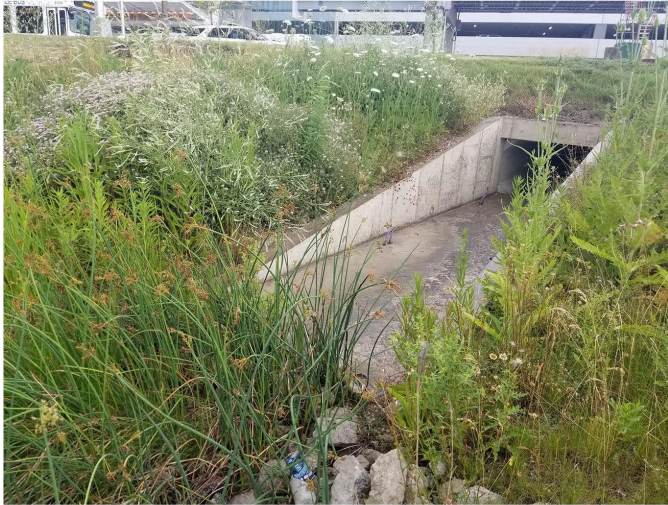
Photo 133. NE19-014, General site, culvert
