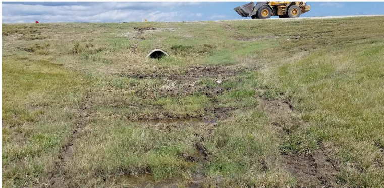
Photo 139. NE19-019, General site, culvert exit. View to the north
