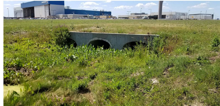
Photo 152. NE19-022, General site, culvert. View to the west
