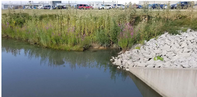
Photo 87. Ditch 30, Inflow culvert
