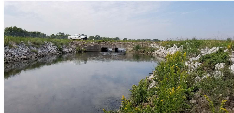
Photo 122. Higgins Creek - Section 2, General site, View to the north
