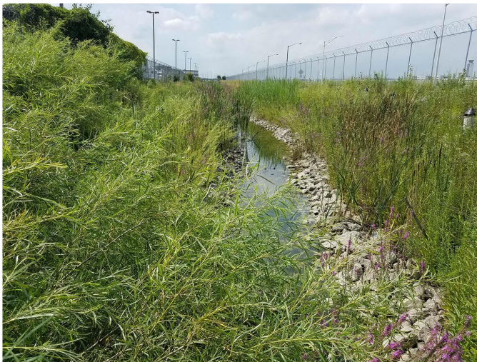
Photo 111. Ditch 43, General site, View to the west
