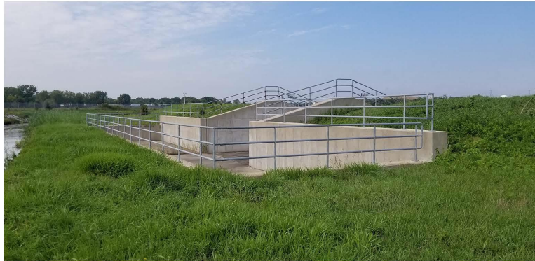
Photo 121. Higgins Creek - Section 1, Higgins Creek spillway. View to the north
