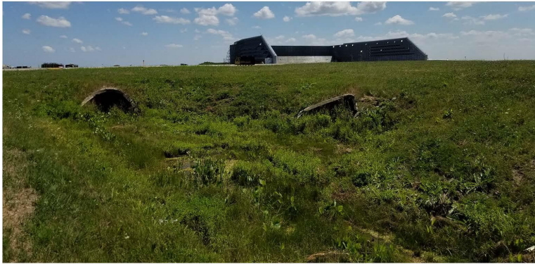
Photo 153. NE19-022, General site, east end culverts View to the southeast
