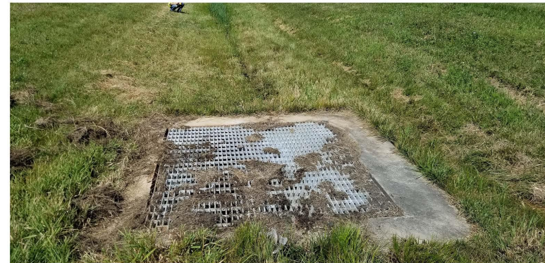
Photo 136. NE19-016, General site, inlet. View to the west
