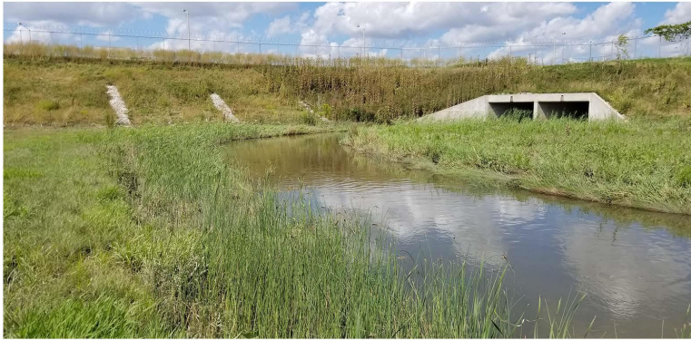
Photo 477. Willow Creek - Section 3, General site, View to the north
