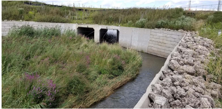
Photo 473. Willow Creek - Section 2, General site, north box culvert. View to the north
