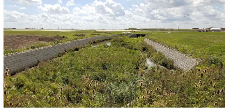
Photo 470. Willow Creek - Section 2, General site, View to the south
