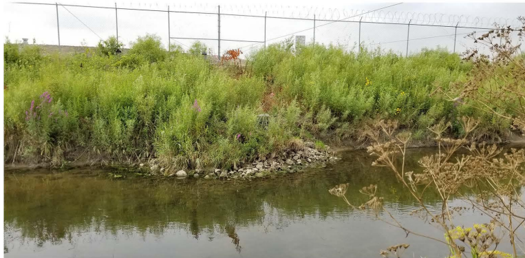
Photo 487. Willow Creek - Section 6, General site, culvert entrance. View to the south
