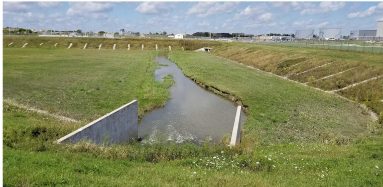
Photo 475. Willow Creek - Section 3, General site, View to the north
