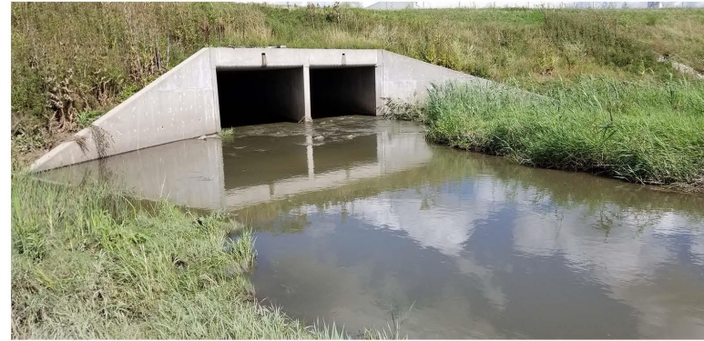
Photo 478. Willow Creek - Section 3, General site, box culvert. View to the north
