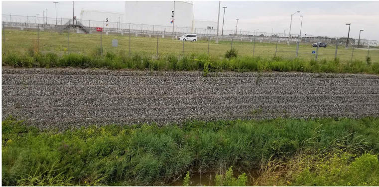
Photo 481. Willow Creek - Section 4, General site, gabion wall. View to the west
