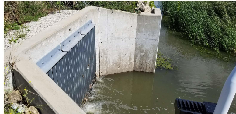
Photo 468. Willow Creek - Section 1, General site, discharge near Middle sister
