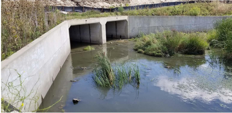
Photo 469. Willow Creek - Section 1, General site, north box culverts. View to the north
