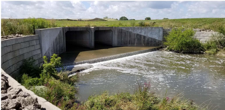
Photo 471. Willow Creek - Section 2, General site, south discharge
