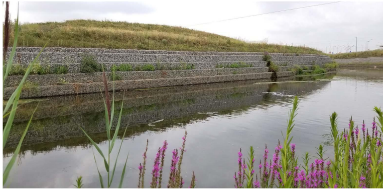
Photo 485. Willow Creek - Section 6, General site, west end gabion wall. View to the west
