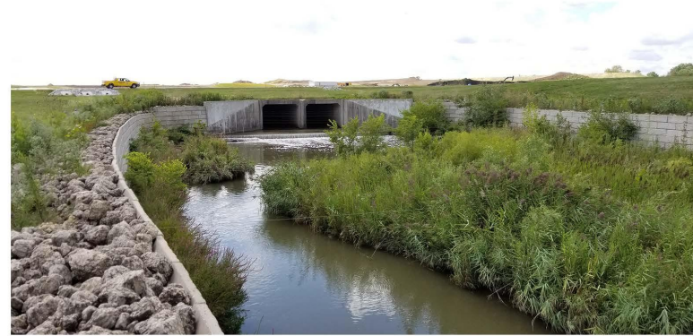
Photo 474. Willow Creek - Section 2, General site, View to the south
