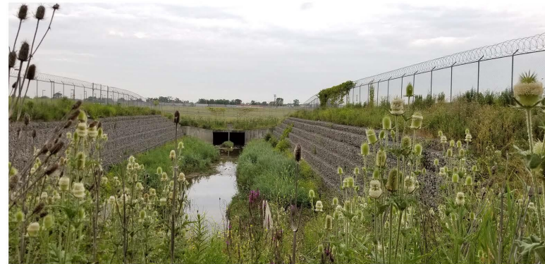
Photo 480. Willow Creek - Section 4, General site, View to the north
