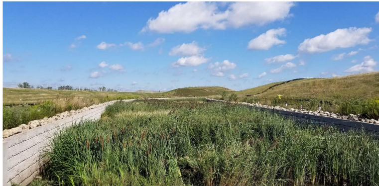
Photo 467. Willow Creek - Section 1, General site, View to the north
