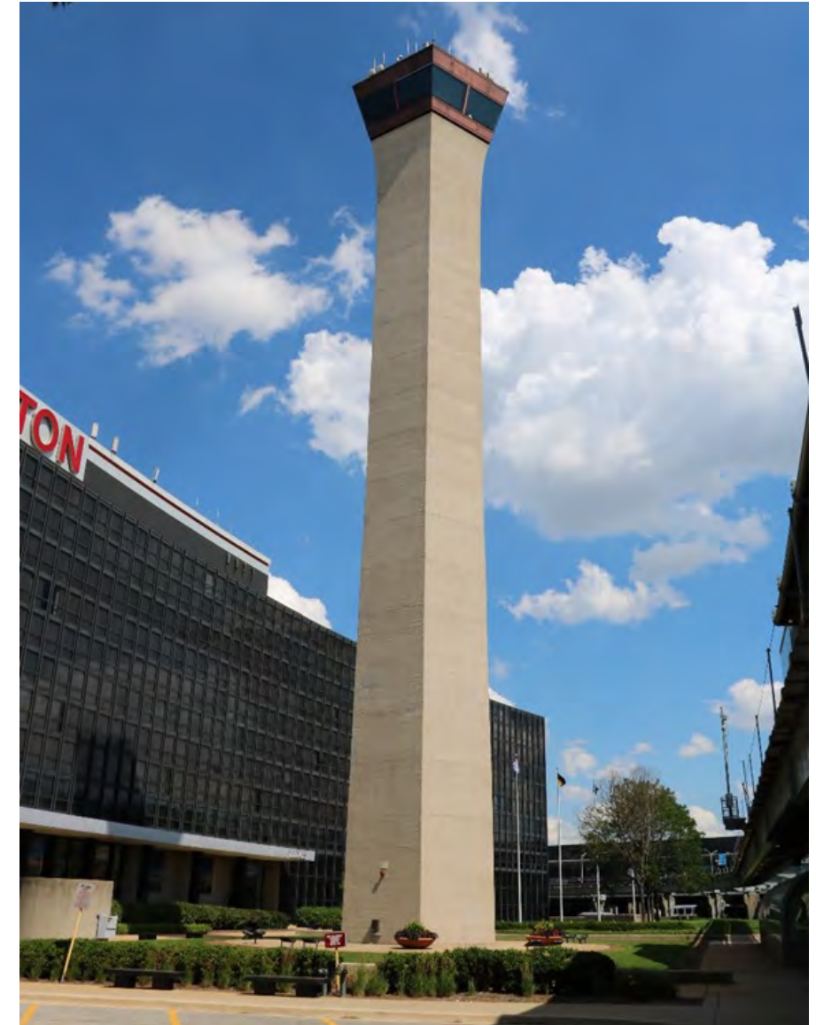
CDA Control Tower
