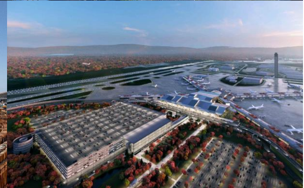
PIT New Terminal
