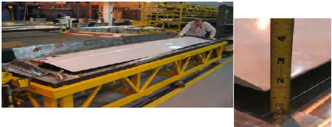
Figure 13: Repaired metallic structure not conforming to geometry
