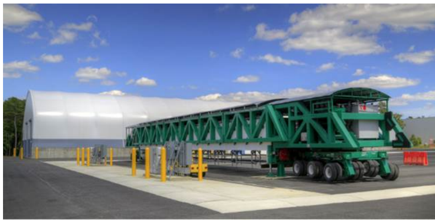
Figure 26: National Airport Pavement and Materials Research Center
