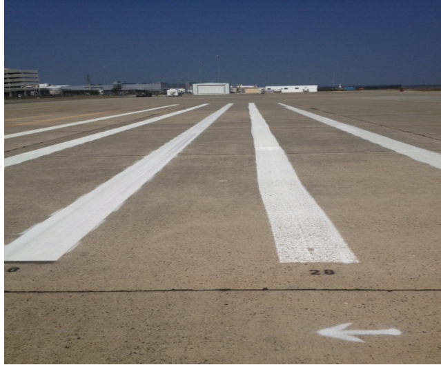
Figure 30: Structural Methyl Methacrylate Paint Markings on Runway
