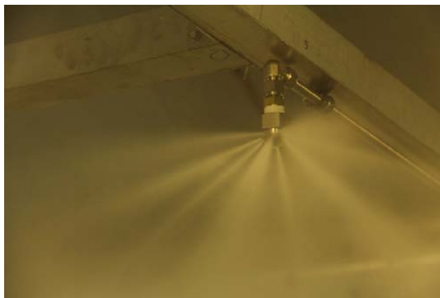
Figure 74: Water Mist Nozzle
