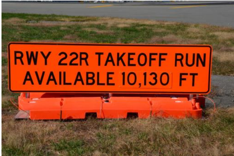
Figure 29: Airport Construction Sign –RWY 22R Takeoff Run Available 10, 130 ft.
