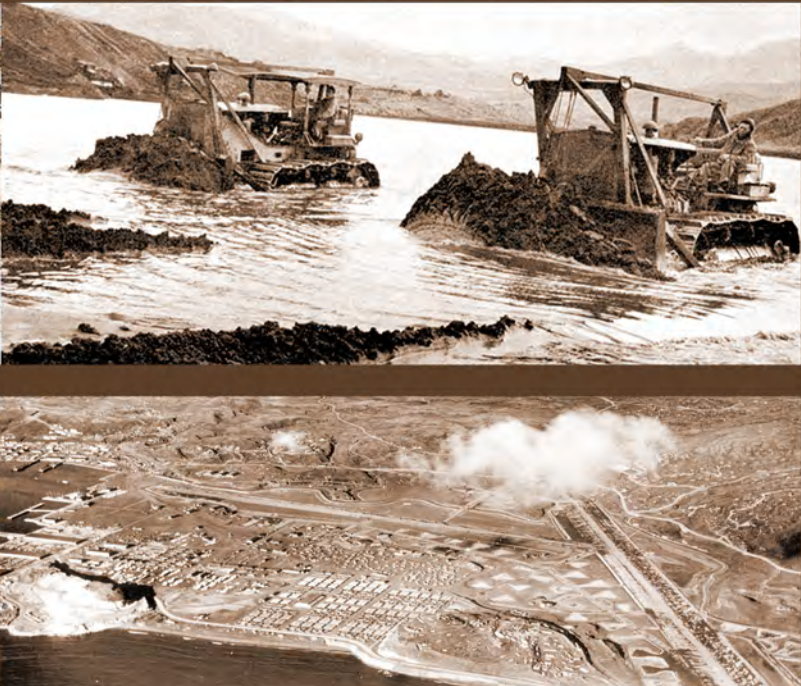
(Top) U.S. Army Engineers dredging tidal flat to create runway at Adak, September, 1943 (www.ww2db.com photo) (Bottom) Adak Army Airfield, WWII (FAA Archives)
