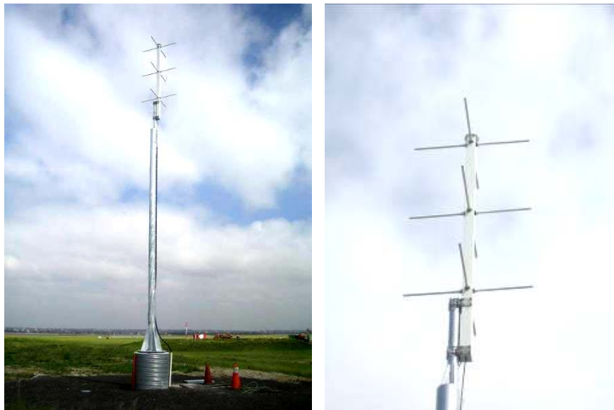
Figure 6 – VHF Data Broadcast (VDB) Antenna
