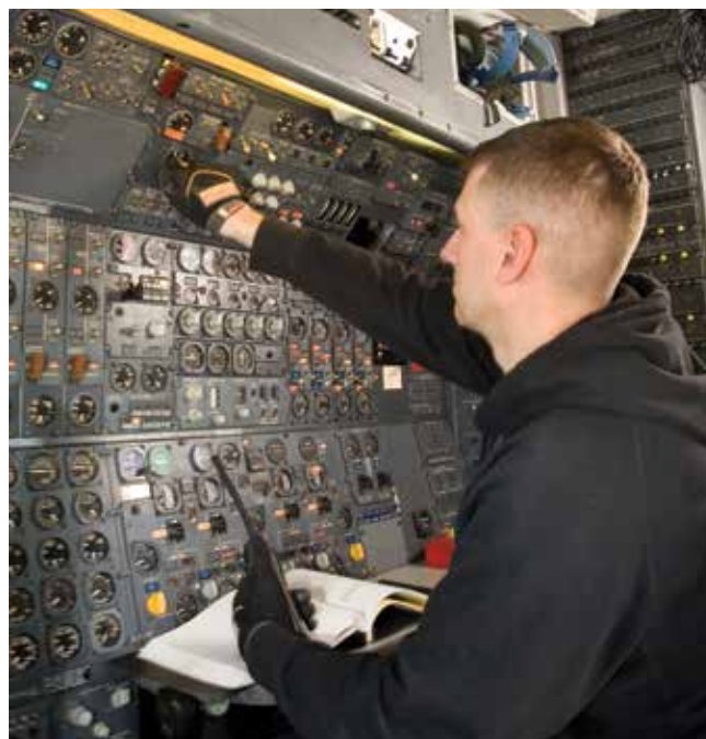
Cargo compartment smoke-detection testing. Photo: FAA.
