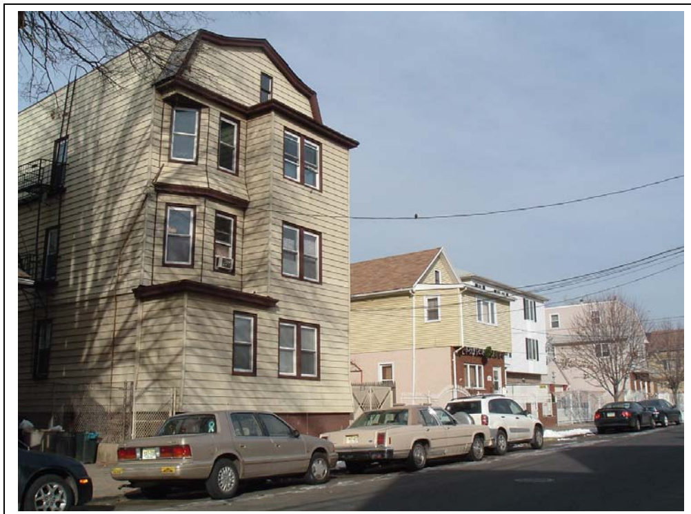
Plate 10: 217 Delaware View: Looking NW Elizabeth, NJ
