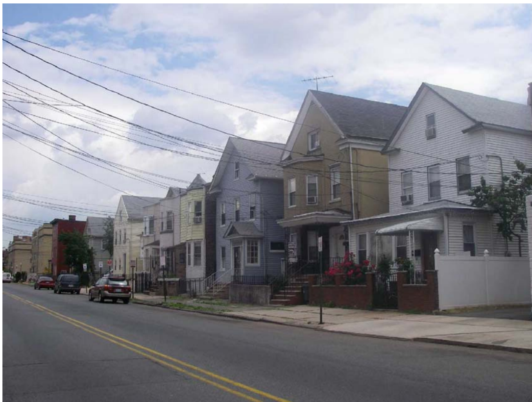
Plate 9: 850–822 E. Jersey St. View: Looking SE
