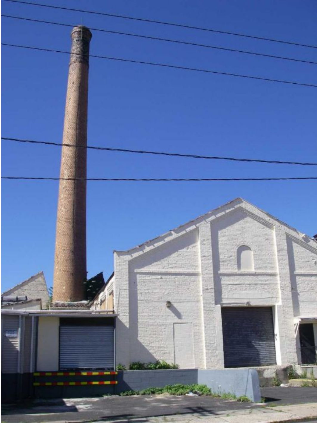
Magnolia AVe ad Division Street 2
