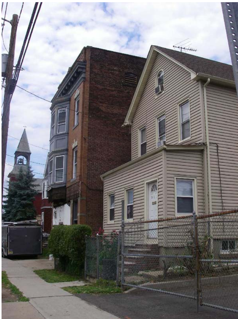
Plate 2: L-R: 953, 947-45, 943, 941 E Grand St. View: Looking NW
