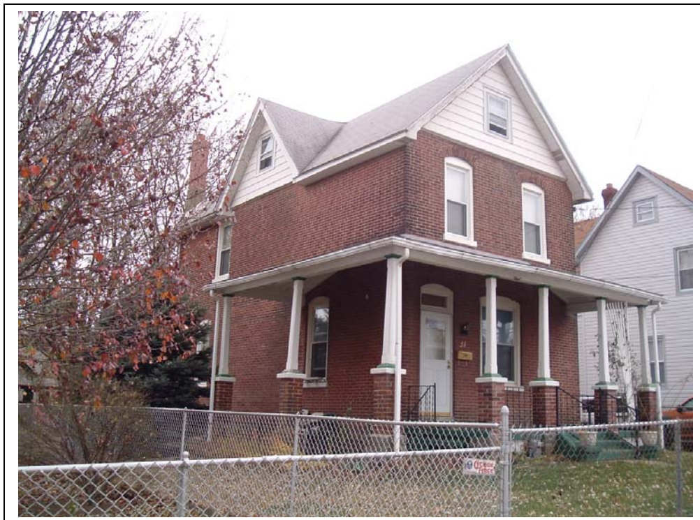
Plate 24: 311 Massasoit St. View: Looking S (N elevation)
