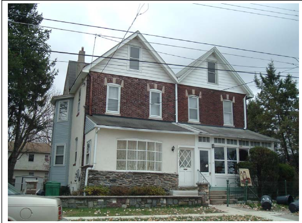
Plate 23: 439 Manhattan St. View: Looking N (S elevation)
