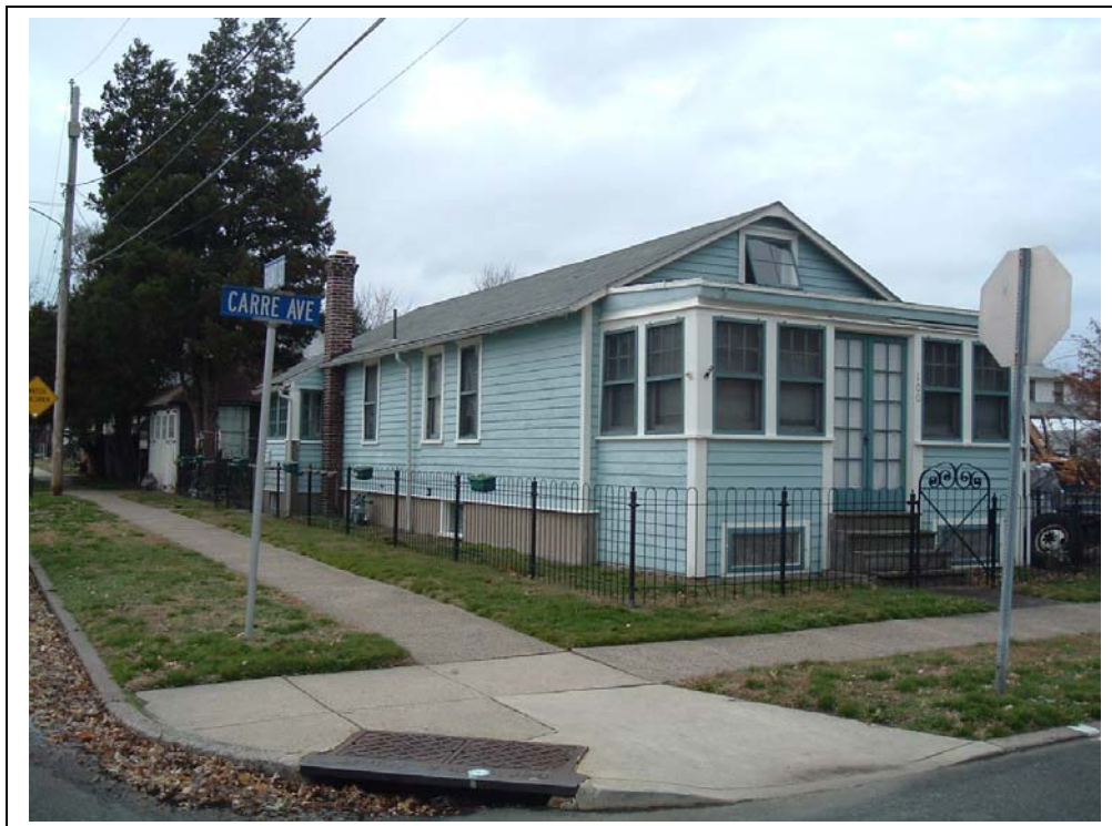
Plate 20: 100 Carre Ave View: Looking NW (S & E elevations)
