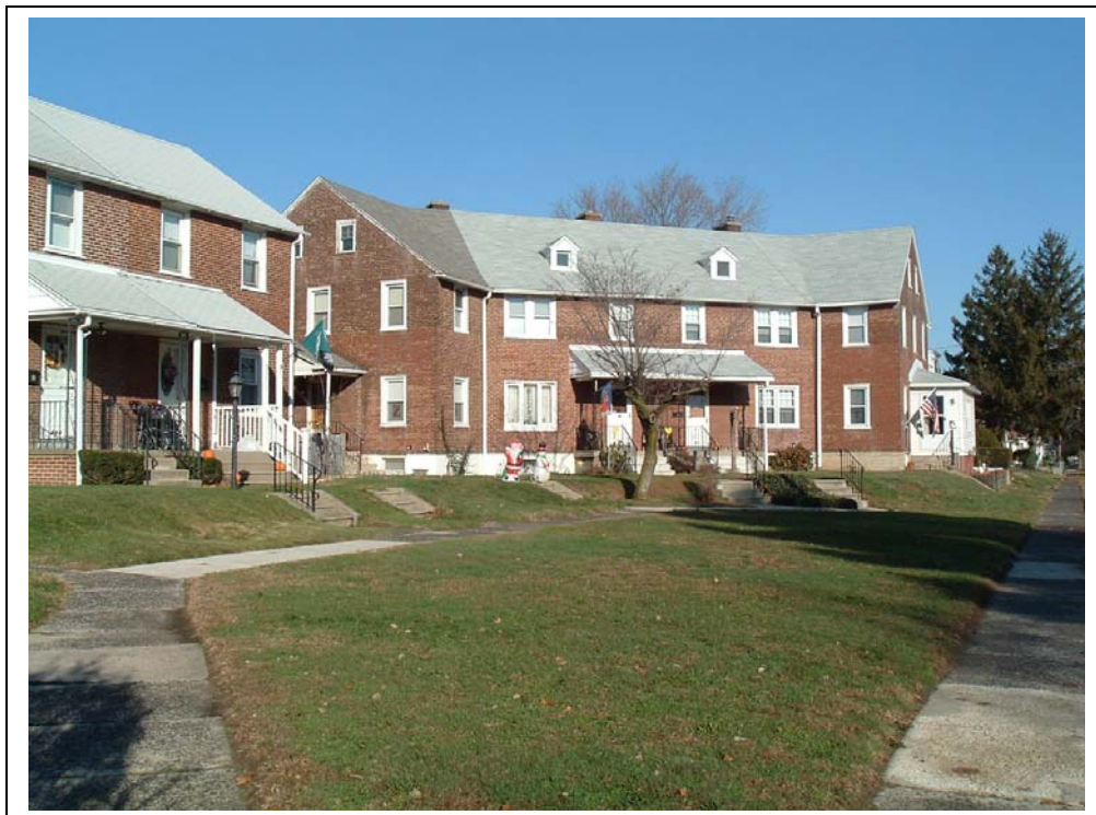
Plate 12: Westinghouse Village (NR eligible district) 535 Jansen Ave. View: Looking NW 045-TI-005
