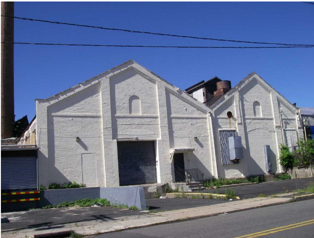
Magnolia Ave ad Division Street 1
