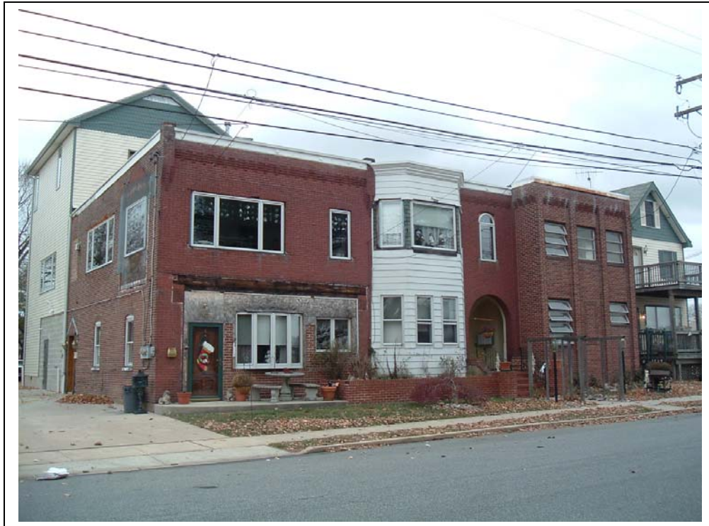
Plate 29: 107 W. 2 nd St. View: Looking NE (W & S elevation)
