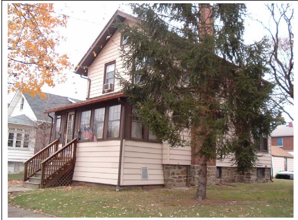
Plate 21: 216 Taylor Ave. View: Looking NE (W & S elevations)
