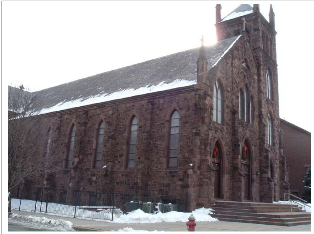
Plate 3: Sacred Heart Church (NR-eligible) Spring & Bond Sts. View: NE & NW elevations Elizabeth NJ
