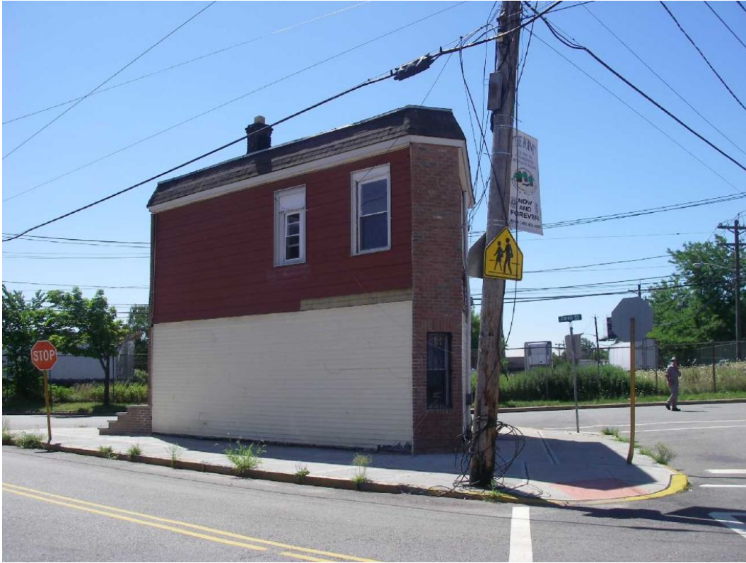
Looking S. New Pt Rd Court and 5th Sts
