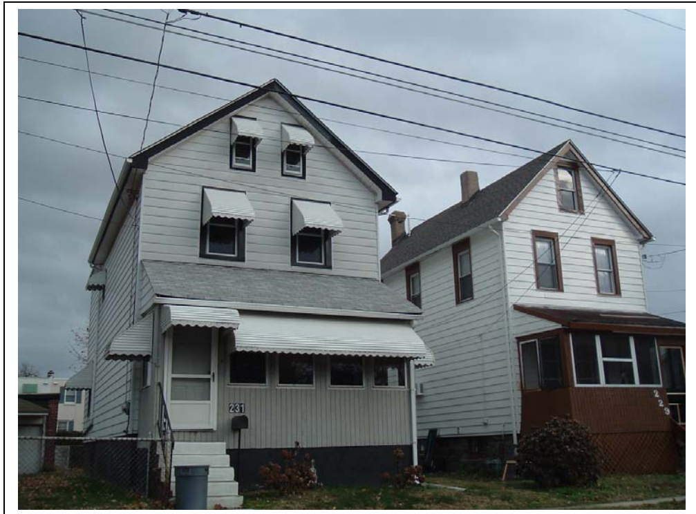
Plate 22: 231 Bartram Ave. View: Looking E (W elevation)
