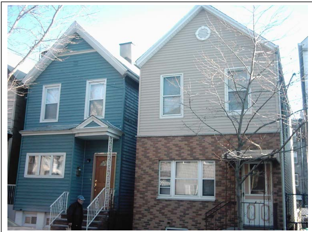
Plate 14: 81 Ann St. View: NW elevation Newark, NJ
