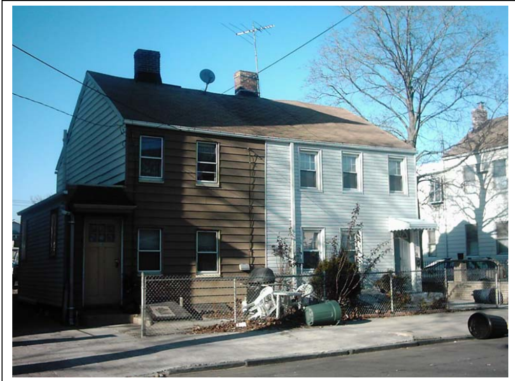
Plate 11: 14 Houston St. View: SE elevation Newark, NJ
