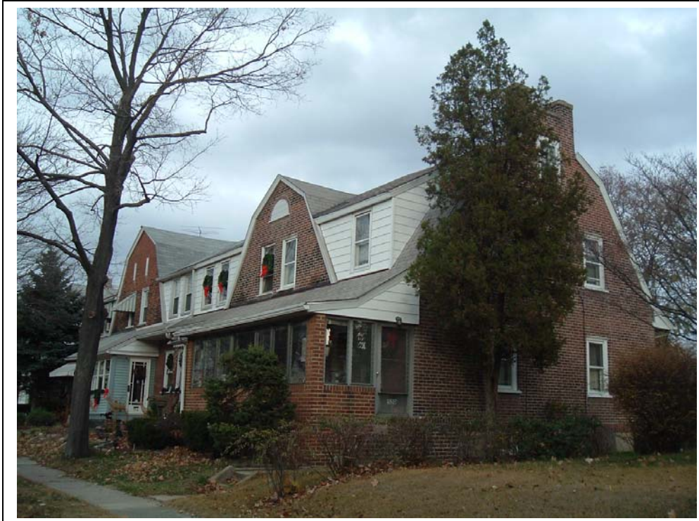
Plate 13: Westinghouse Village View: 550 Saude Ave View: Looking NE
