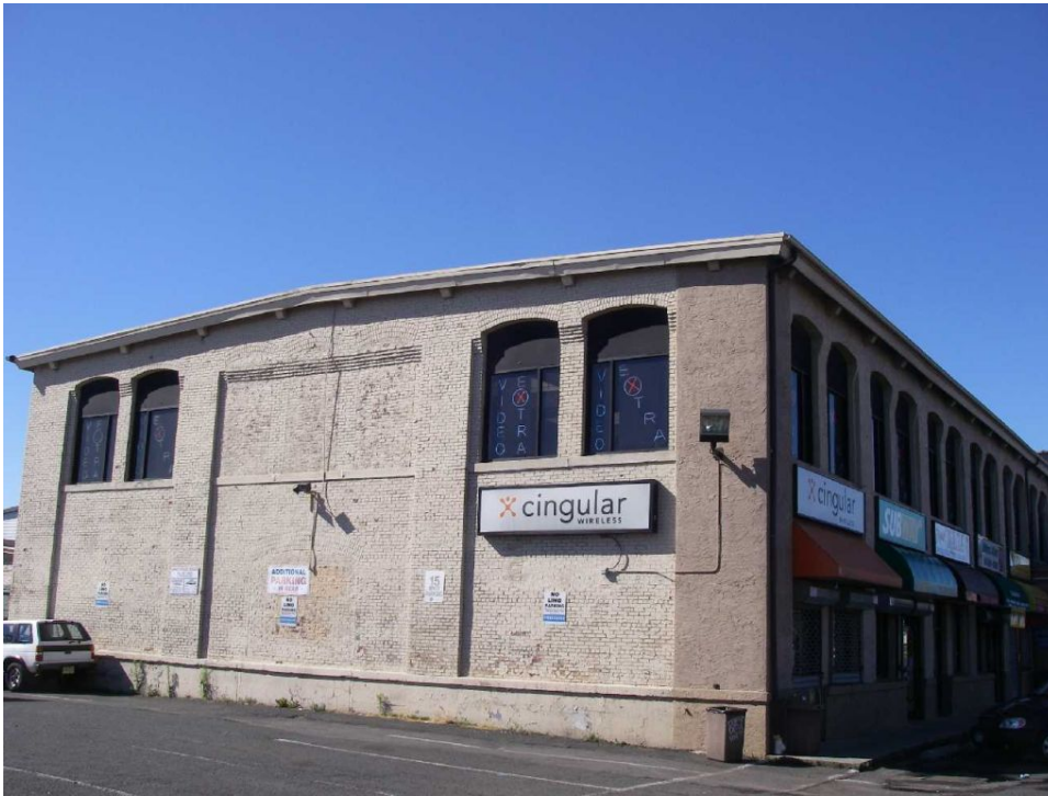
Hitching Building Spring Street
