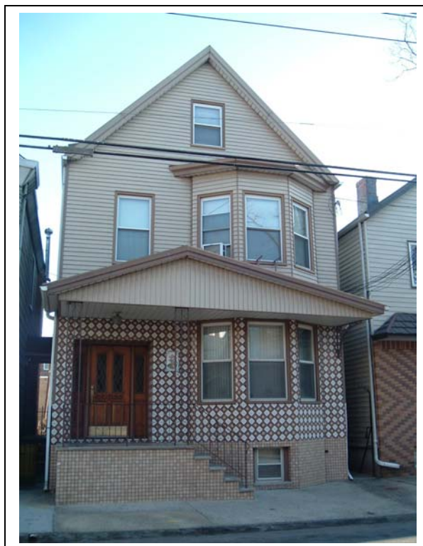
Plate 8: 37 Napoleon St. View: NW elevation Newark, NJ
