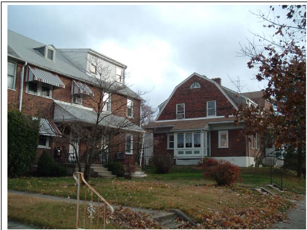
Plate 14: Westinghouse Village 544 Saude Ave. View: Looking SE
