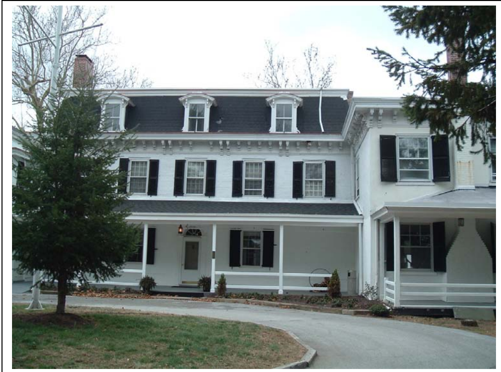
Plate 3: Corinthian Yacht Club (NR eligible) PHMC #079244 View: Looking S (N elevation) 045-TI-001
