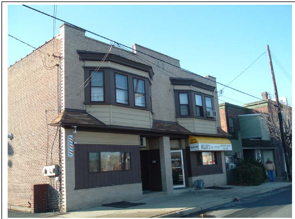
Plate 30: 6 W. Powhattan St. View: Looking SW (E & N elevations)
