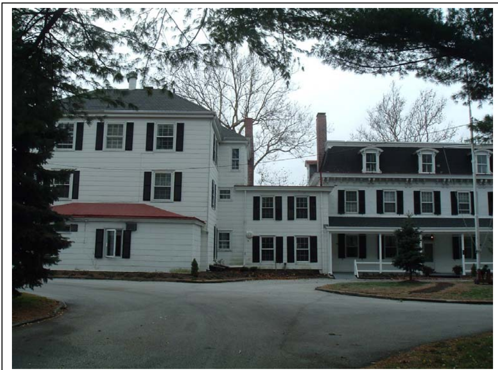
Plate 4: Corinthian Yacht Club View: Looking S (N elevation)
