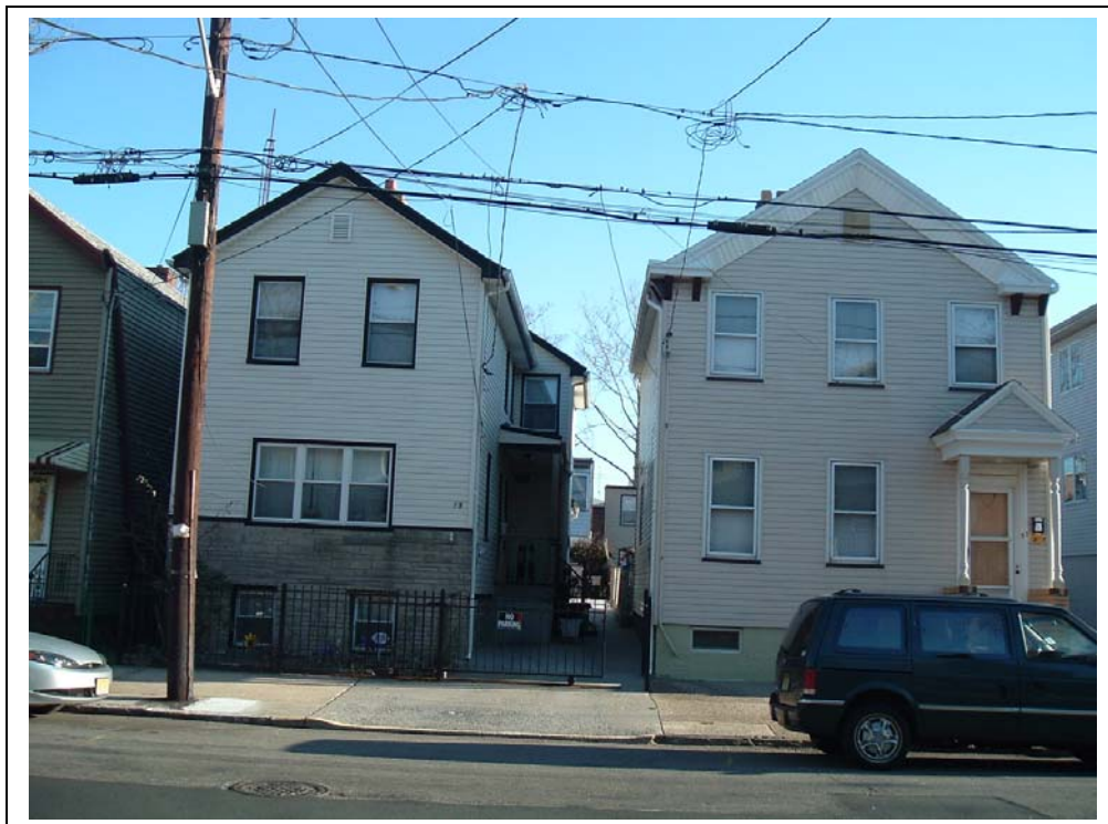
Plate10: 19, 17 Napoleon St. View: NW elevations Newark, NJ
