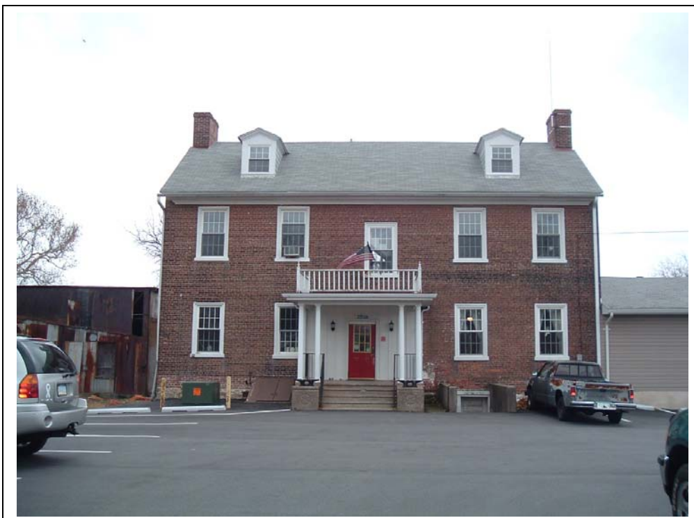
Plate 8: The Lazaretto: Physicians' Residence View: Looking S (N elevation)
