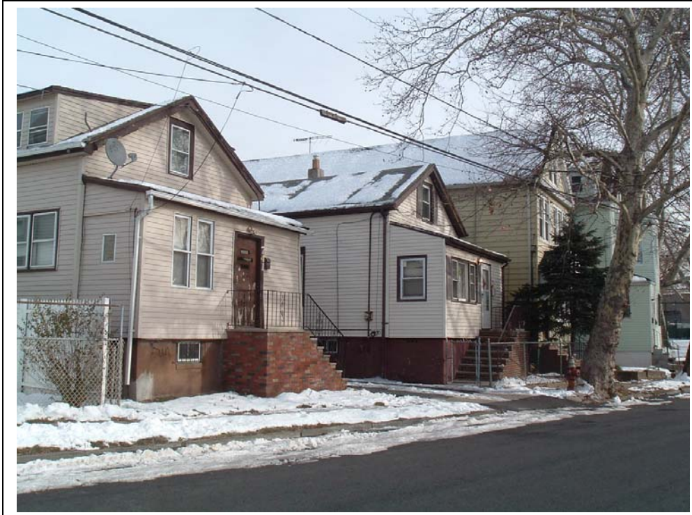
Plate 7: 741 S. Park St. View: Looking NE Elizabeth, NJ
