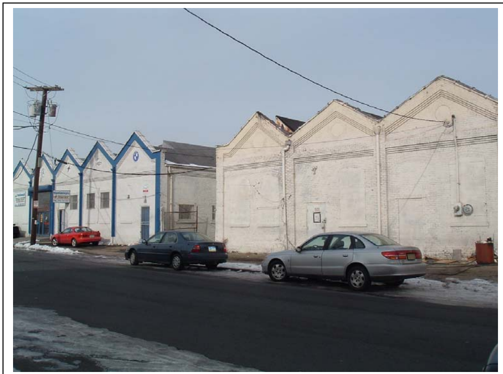
Plate 6: 801 Magnolia: near CRRNJ View: SW elevation Elizabeth NJ
