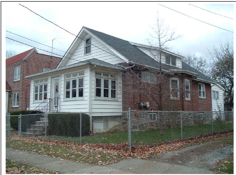
Plate 18: 218 Taylor Ave. View: Looking NE (W & S elevations)
