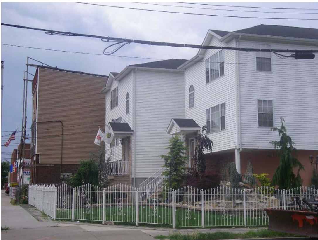
Plate 14: 601-5 E. Jersey St. View: SW & SE elevations
