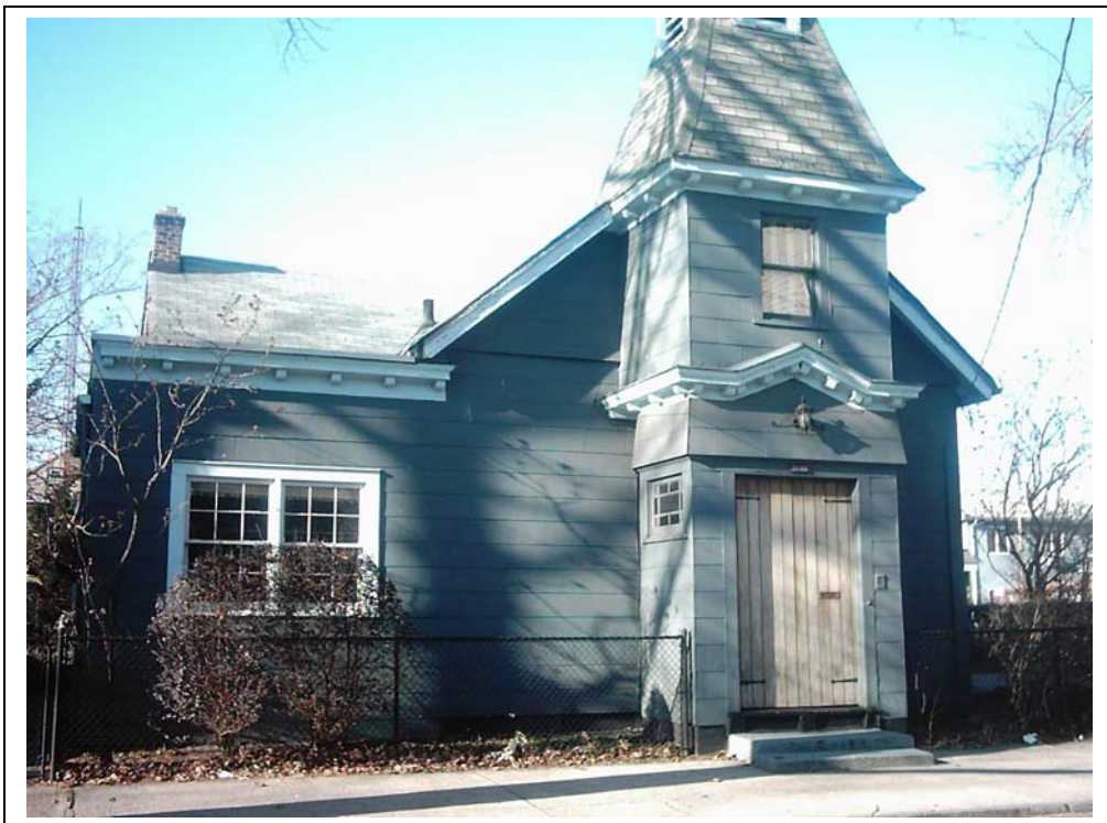
Plate 12: 26-30 Houston St. View: SE elevation Newark, NJ
