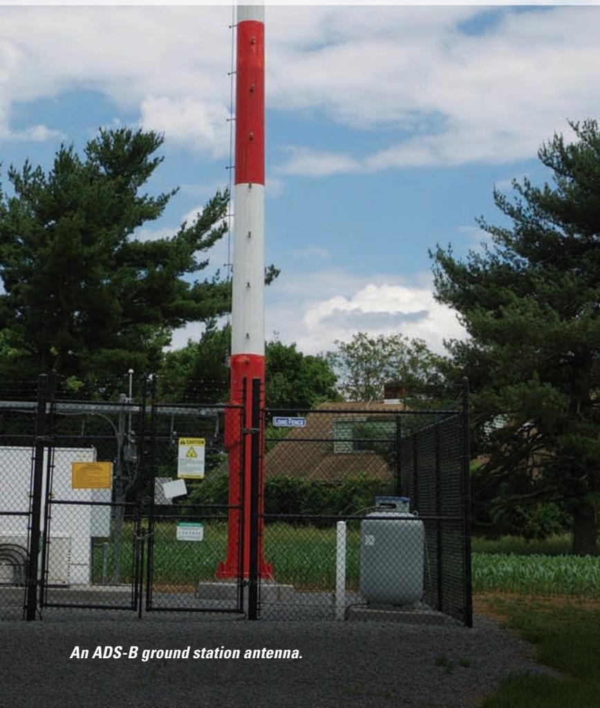
*An ADS-B ground station antenna.*
