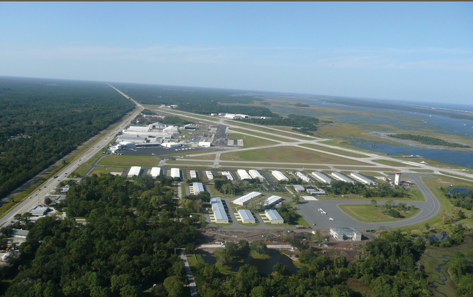
Aerial view of NFRA from the south side of the airport.
