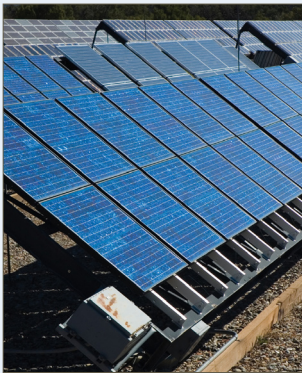
Example of a Solar PV array.
