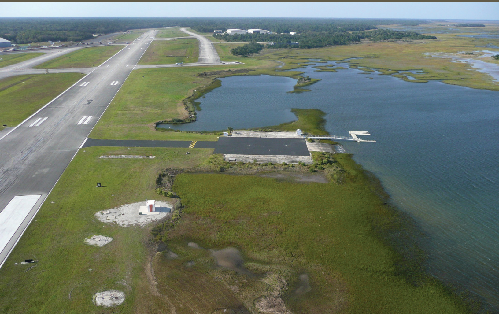
✈ NFRA's seaplane ramp and lanes.
