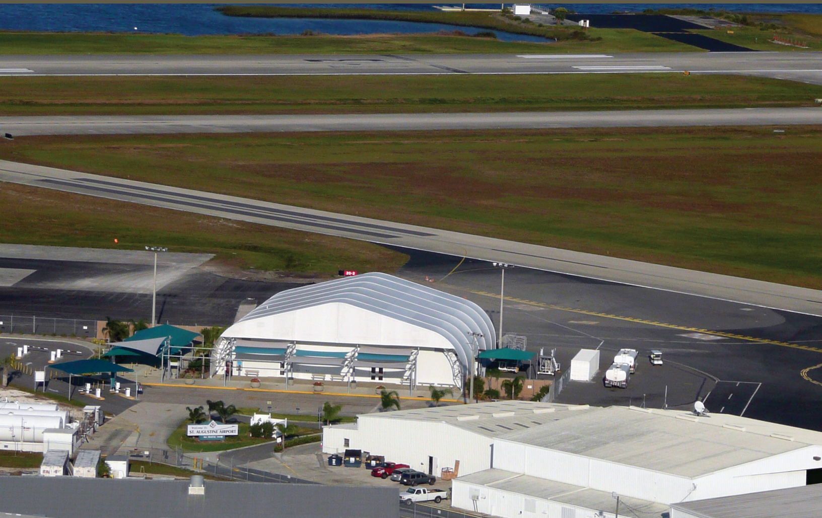
✈ Airport passenger airline terminal and tenant facilities.
