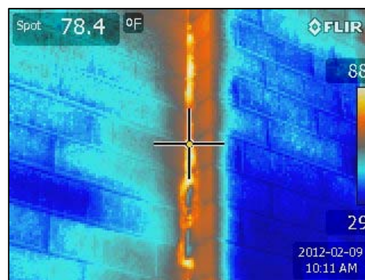
Typical results of an infrared (IR) imaging study. Orange areas in the photo on the right indicate gaps in the building façade where warm air is leaking out.
