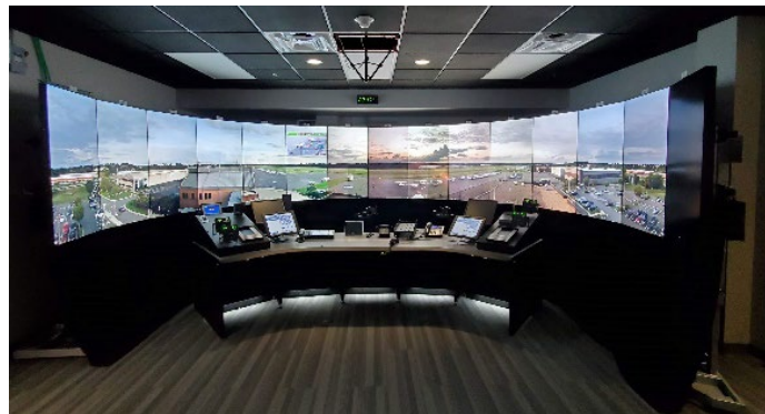
Remote Tower Module (Equipment, console, and displays)
