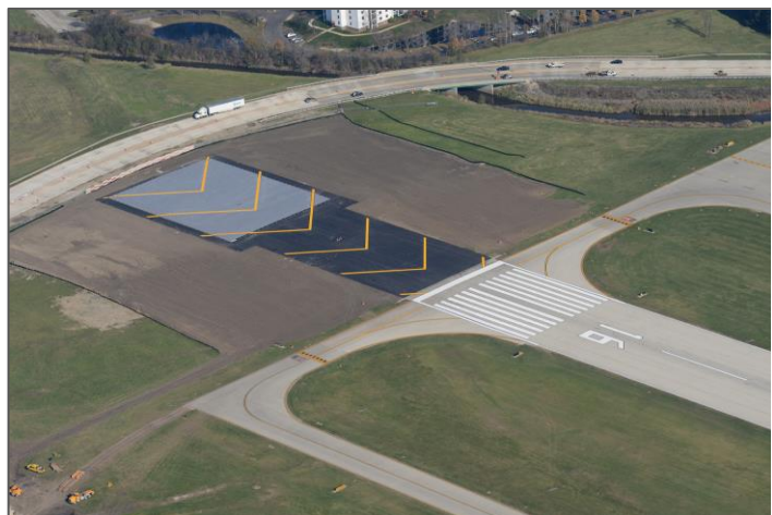
Figure 5: EMAS on the Approach End of Runway 16 at Chicago Executive Airport, IL
