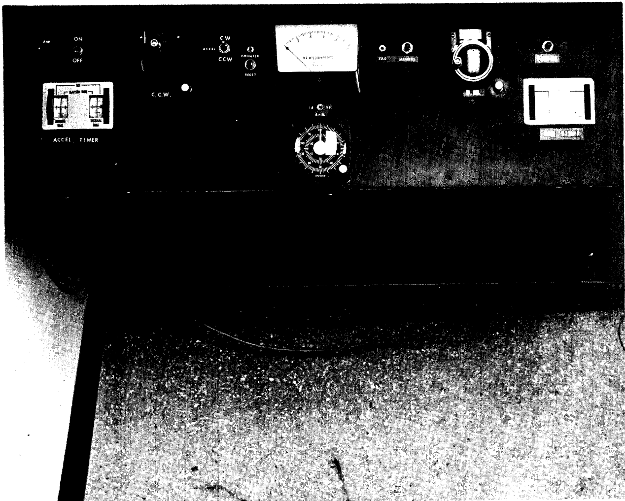
FIGURE 5. View of control panel.
