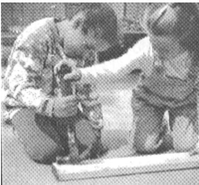
1st - Using a level
