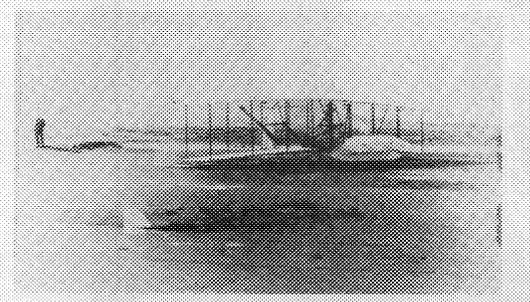
*The fourth flight was the longest -852 feet in 59 seconds - with Wilbur Wright at the controls. It also resulted in minor damage to the elevator supports during a hard landing. Shortly after this picture was taken, however, the machine badly damaged by the gusty winds, ending flight testing for the year.*
