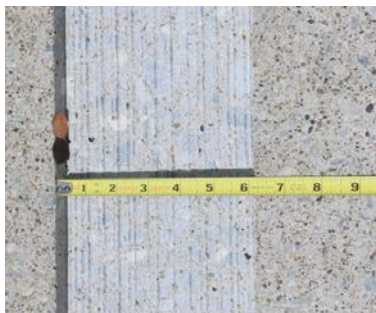
(c) The 6" Wide Sawcut Rumble Strip
