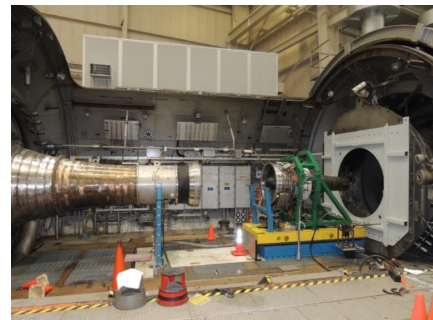
NASA Propulsion Systems Lab Altitude Facility
