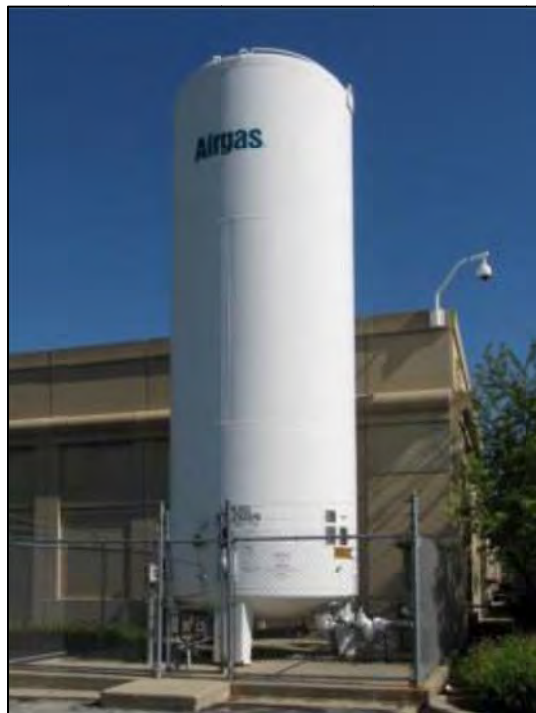
Exhibit 2-3. Typical LOX and LN 2 Storage Tank
