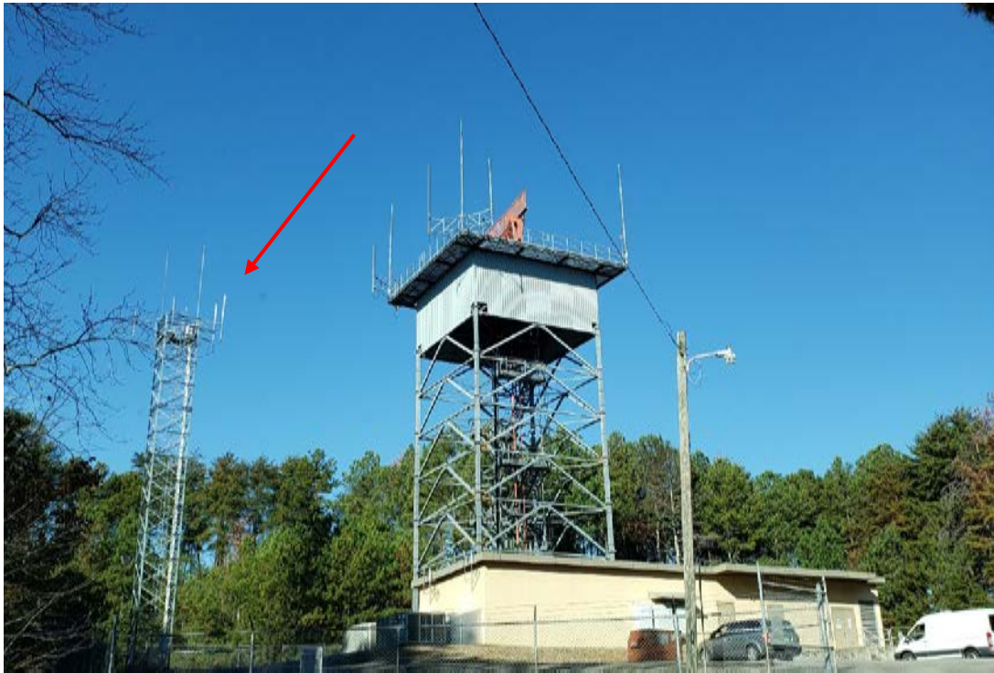
Figure 3. An RTR Collocated with an Airport Surveillance Radar (ASR), with RTR Antennas Indicated
