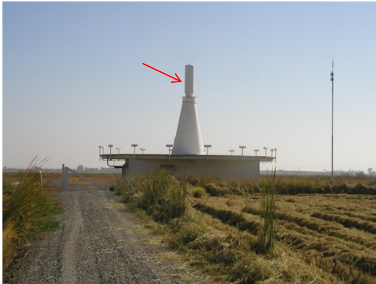
Figure 3-13. VORTAC Station, Showing TACAN Antenna on Top
