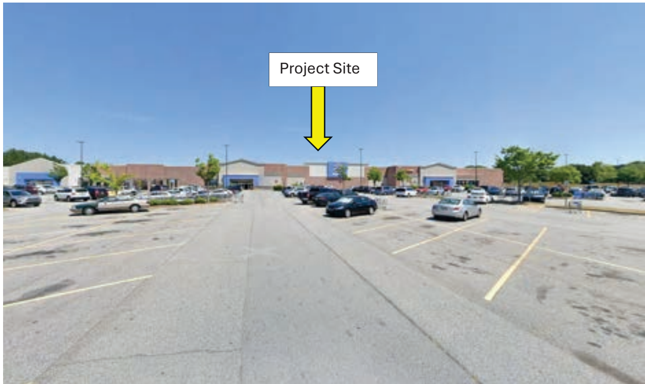
3435 Centerville Hwy Snellville GA 30039 nest site, view north. Google Street View, 2022.
