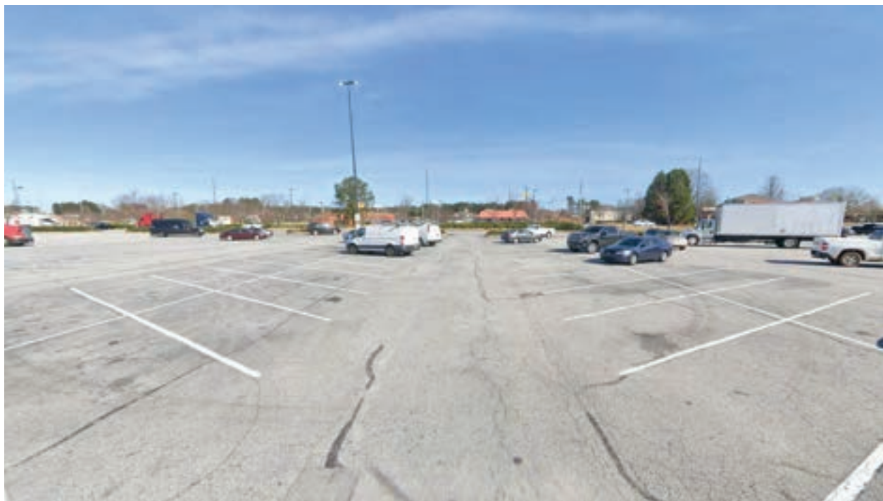
1025 GA-34 Newnan GA 30265 nest site, view north. Google Street View, 2022.
