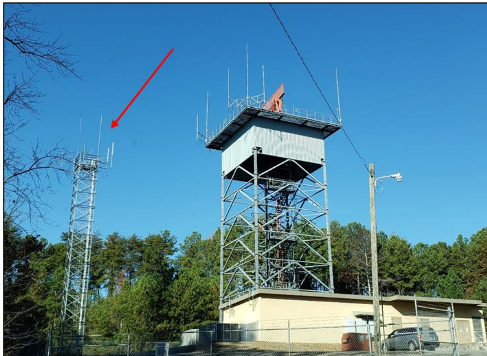
Figure 3: RTR Co-Located with ASR
