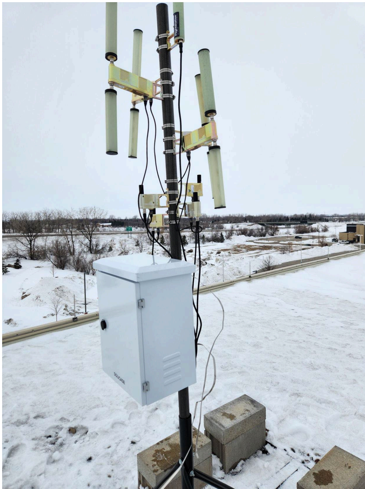
Figure 18: uAvionix SkyStation-5060 POE GRS Installed on the Roof of the NPUASTS Tech Accelerator Building.
